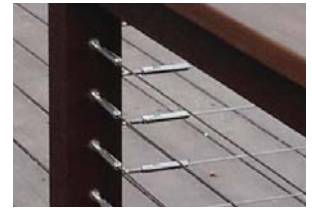
Wood cable system with Adjustable Bodies
