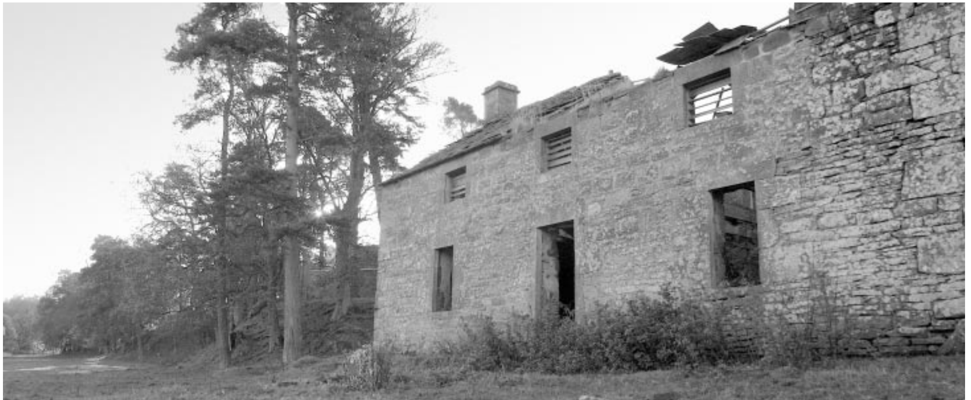
Part of Kincaldrum Mill buildings.
