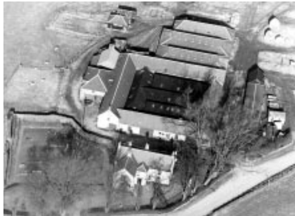
Aerial view of the Mill of Inverarity prior to demolition.
