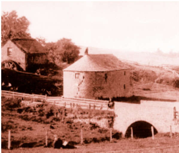
The mill at Holemill in 1888, when the waterwheel was still present.
