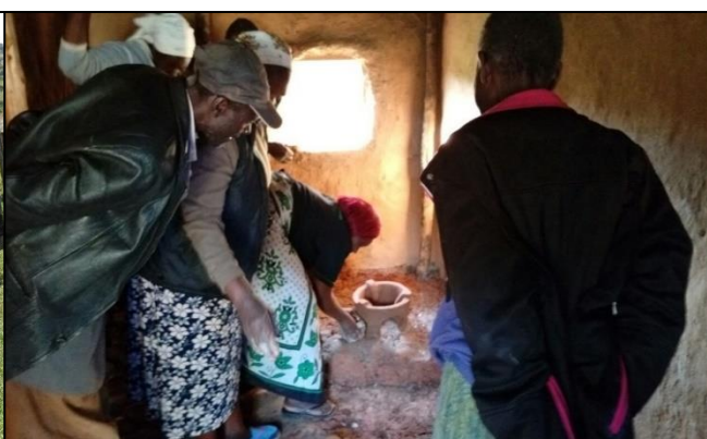
Demonstration on the construction of the Kuni Mbili Jiko in Kapsait, Elgeyo Marakwet County
