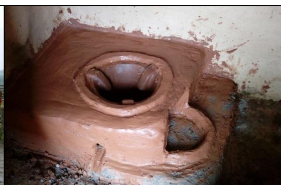
A complete Kuni mbili jiko constructed at Kaptek, Elgeyo Marakwet County
