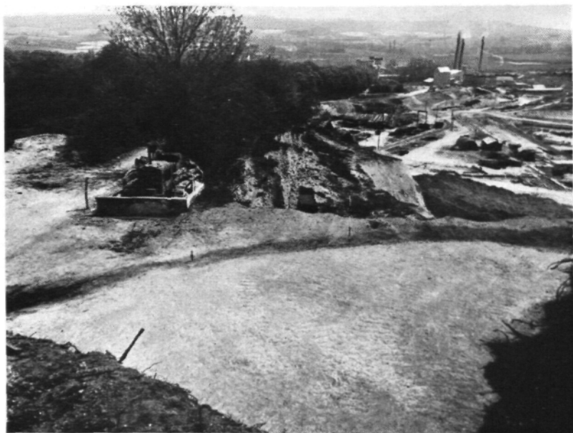
(b) N.E. quadrant removed, showing line of silted ditch
