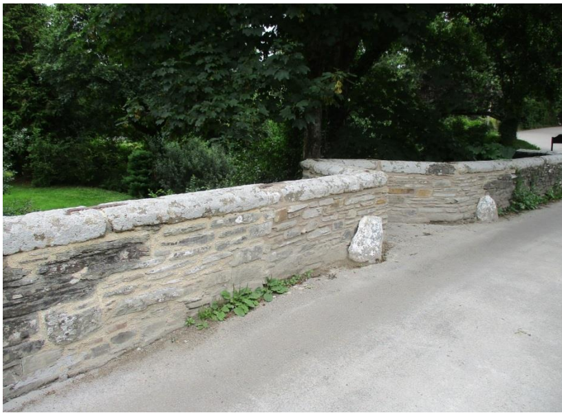
A beautiful repair to the upstream parapet
