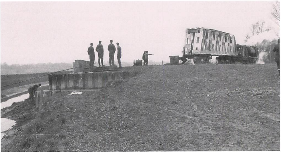
The replacement bridge arrives at Newmill Channel on 11th December 1976 (CSHA)
