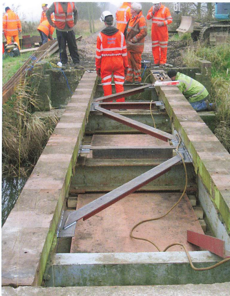
Hexden Bridge with new plan bracing installed (Graham Bessant)
