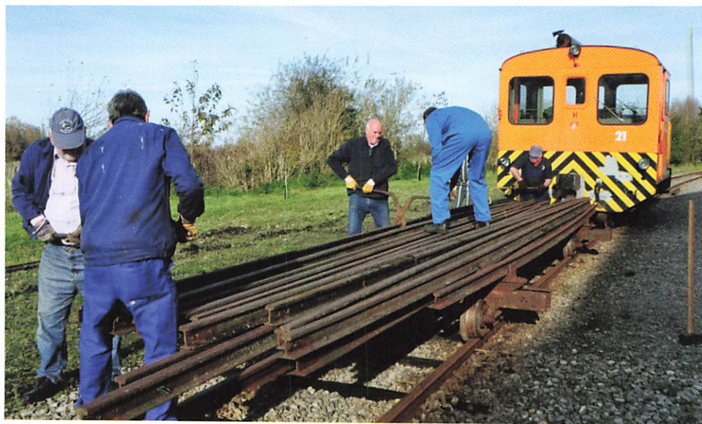
Work gang at Lanchères Pendé (Mike Bunn)
