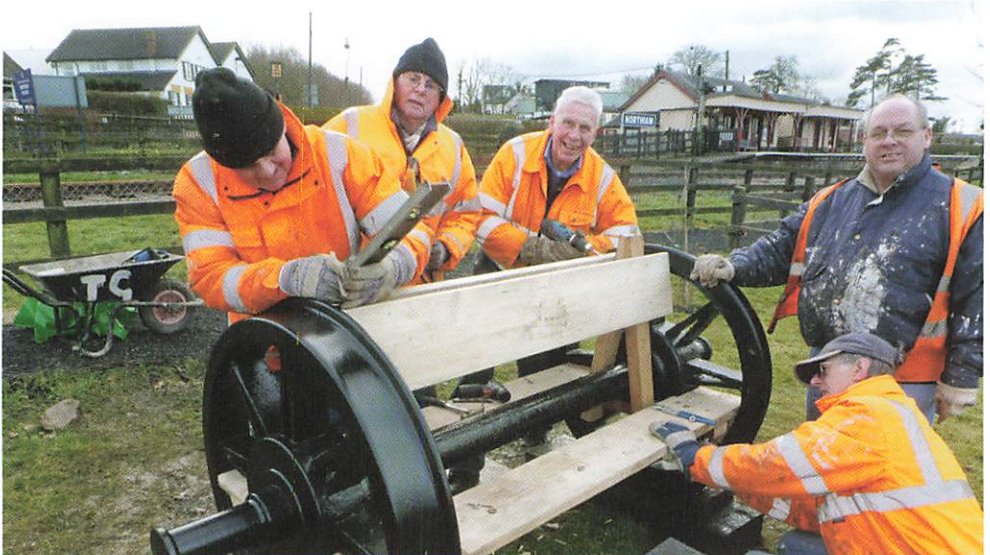
The Tuesday Gang constructing the new seat at Northiam (Humphrey Atkinson)
