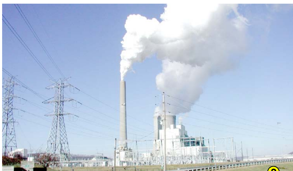
LG&E operates this 566 megawatt coal-fired power plant along the Ohio River just north of Wises Landing in southeastern Trimble County. Photo by Dan Carey, Kentucky Geological Survey.
