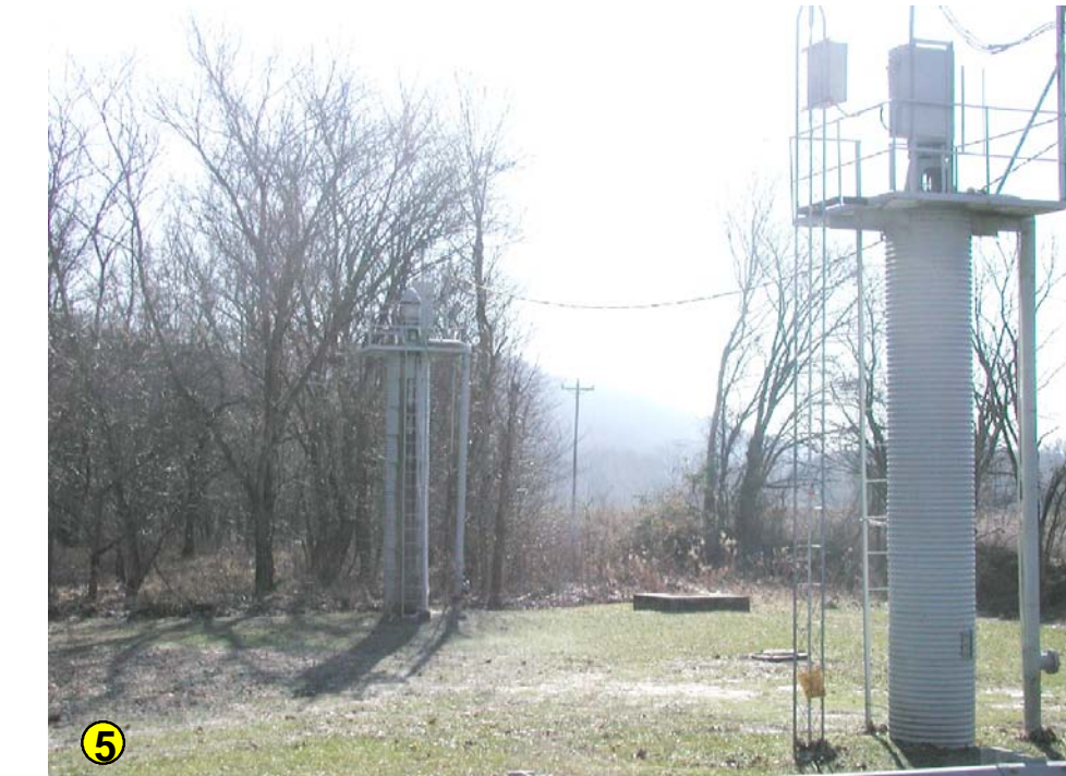
Public water wells in the Ohio River alluvium (unit 1). This aquifer can meet water needs for communities, industry, and power generation. Photo by Dan Carey, Kentucky Geological Survey.
