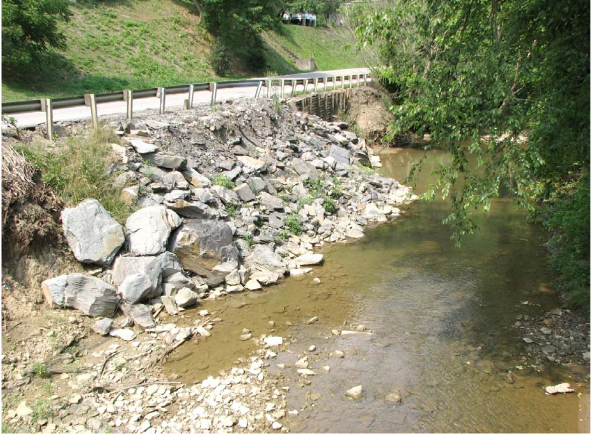
Streambank and pavement support for roadbeds cut into slopes underlain by shale along streams. Photo by Dan Carey, Kentucky Geological Survey.
