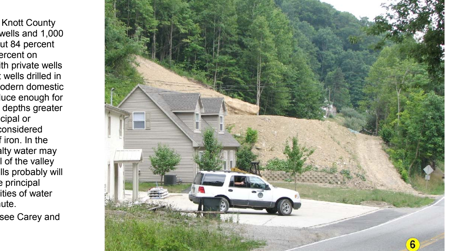
Cut-and-fill foundation preparation is common in steep-sloping areas. Slope stability is maintained by retaining walls and other permanent vegetative covers. See diagram above. Photo by Dan Carey, Kentucky Geological Survey.
