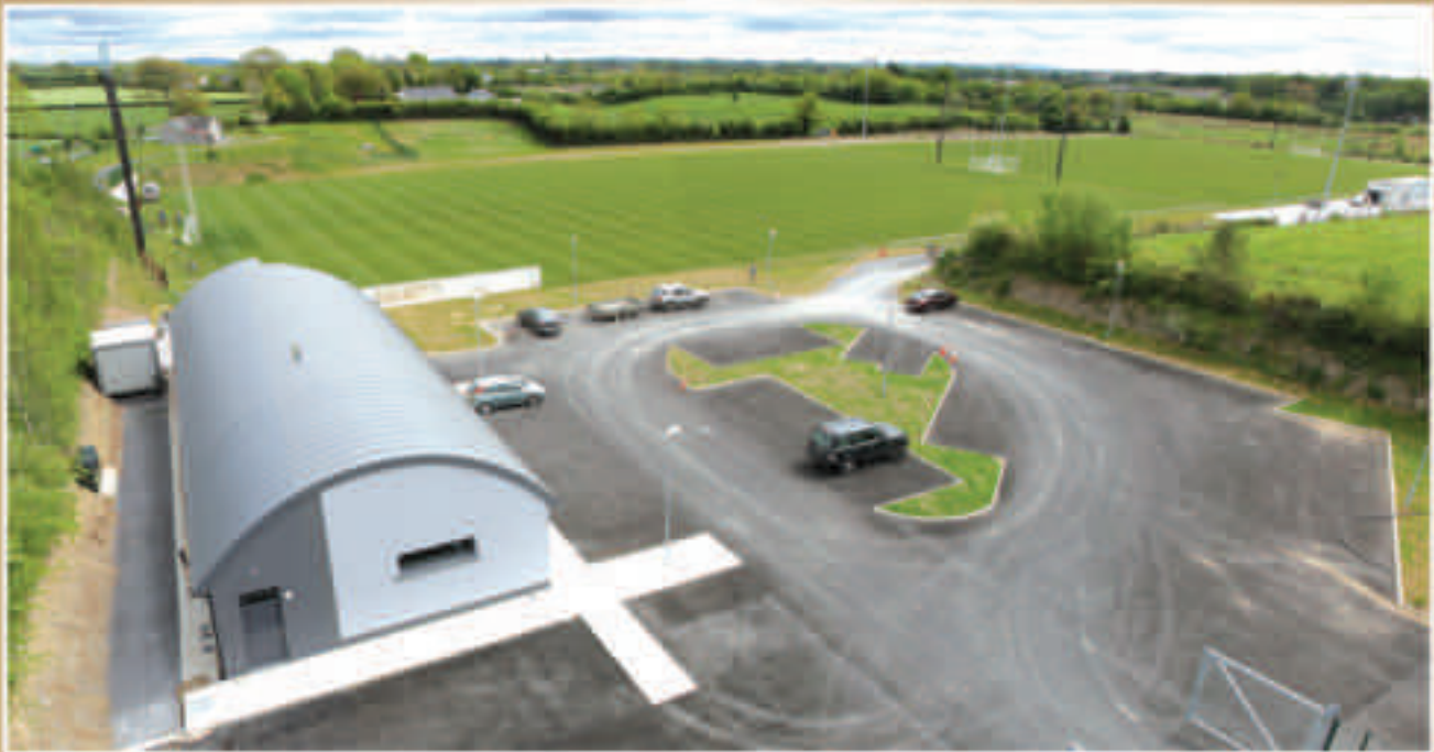
Overhead View of Completed Training Centre at Dunmore (Eoin Hennessy)
