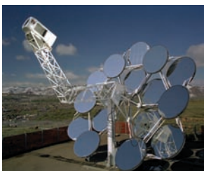
A 25-kilowatt dish/engine solar power system at the National Renewable Energy Laboratory.
