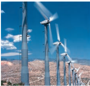
National Renewable Energy Laboratory
