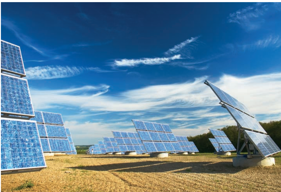
FIGURE 10-9 The Erlasee Solar Park near Arnstein in Bavaria, Germany, is composed of an array of sun-tracking photovoltaic cells that produced a combined power output of 12 MW.
