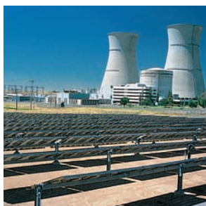
National Renewable Energy Laboratory
