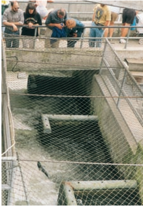
National Renewable Energy Laboratory
