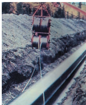
FIGURE 14-6 Zinc wire is attached to this underground pipe at intervals of 500–1000 ft. The zinc loses electrons more easily than the iron and is therefore oxidized instead of the iron.
