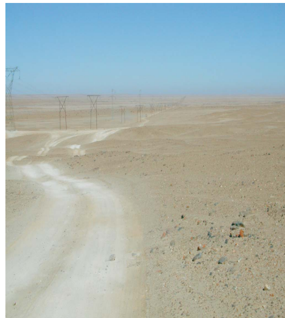
Photo 30: Power-line dissecting the lichen fields of the Naukluft Plateau and destroying the lichen communities along its way due to off-road driving required for service and maintenance.
