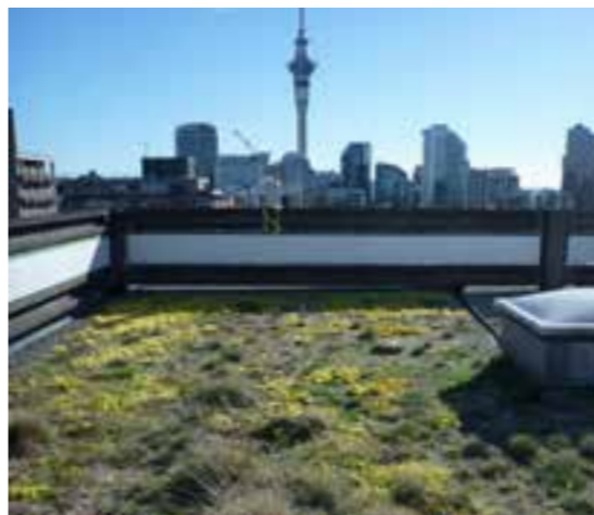
The University of Auckland green roof
