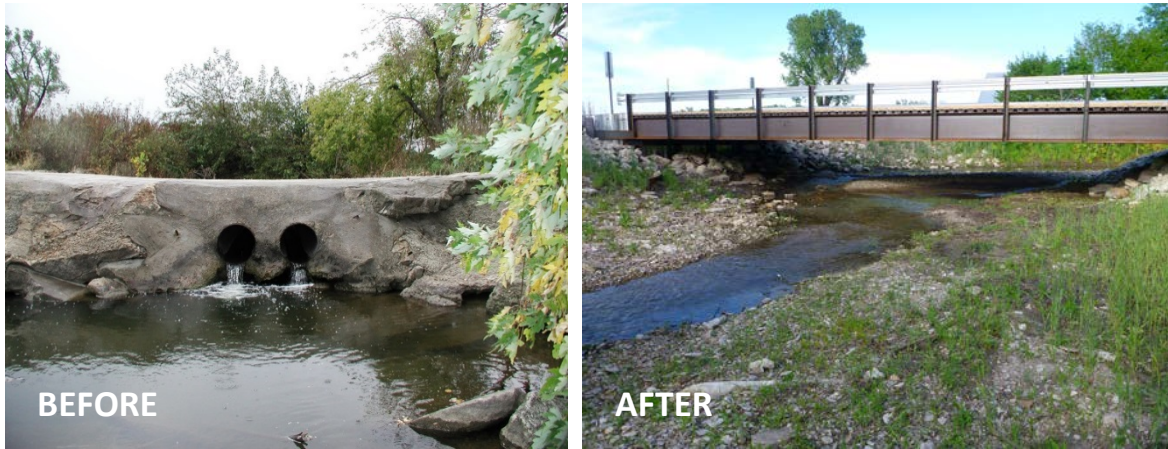
Replacement of perched culverts with a span bridge on Clear Fork Creek, Pottawatomie County
