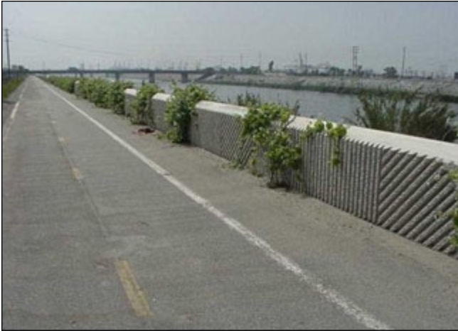
Figure 8.25 Concrete, textured parapet wall along the Los Angeles River in Long Beach
