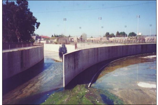
Figure 4.1 Rectangular channel condition at the confluence of Bell and Calabasas Creeks.
