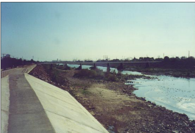
Figure 1.3 Soft bottom portion of Los Angeles River at Willow Street, Long Beach
