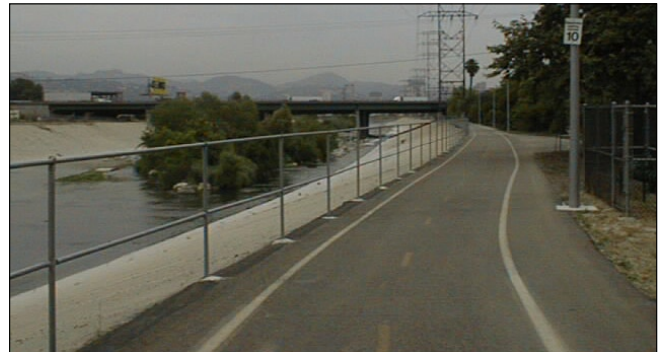
Figure 5.5 City of Los Angeles Bike Path, west bank, fencing on trapezoidal channel
