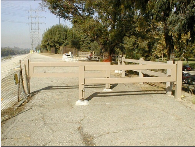
Figure 14.17 Custom steel swing gate designed and installed by North East Trees at Los Feliz Boulevard for equestrians.
