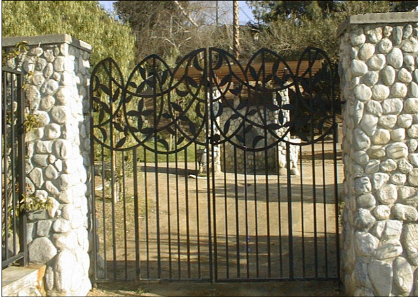
Figure 14.4 Custom wrought iron gate used in conjunction with tubular steel fence. Installation to be done in accordance with manufacturers specifications.
