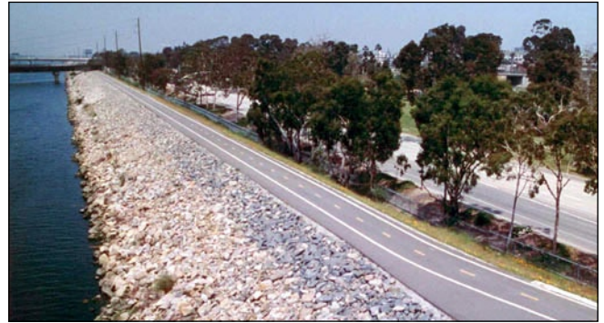
Figure 5.4 Los Angeles River Bike Path, no fencing on trapezoidal channel
