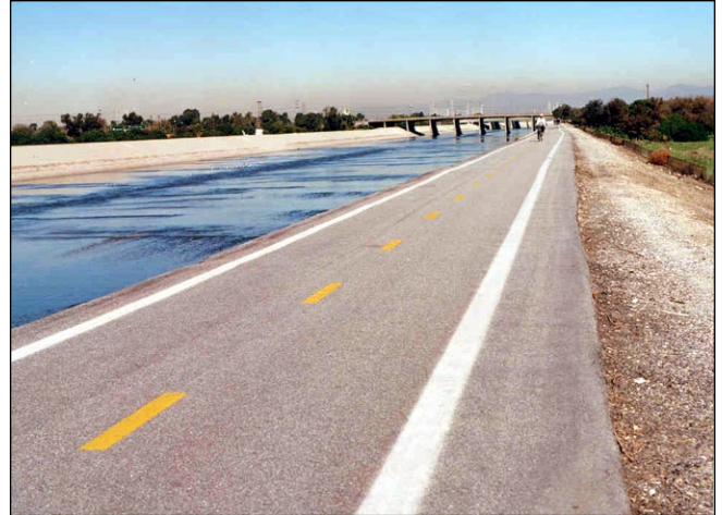
Figure 4.7 Leveed trapezoidal condition in Long Beach
