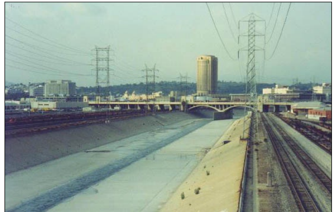
Figure 4.2 Entrenched trapezoidal condition at Fourth St. Bridge.
