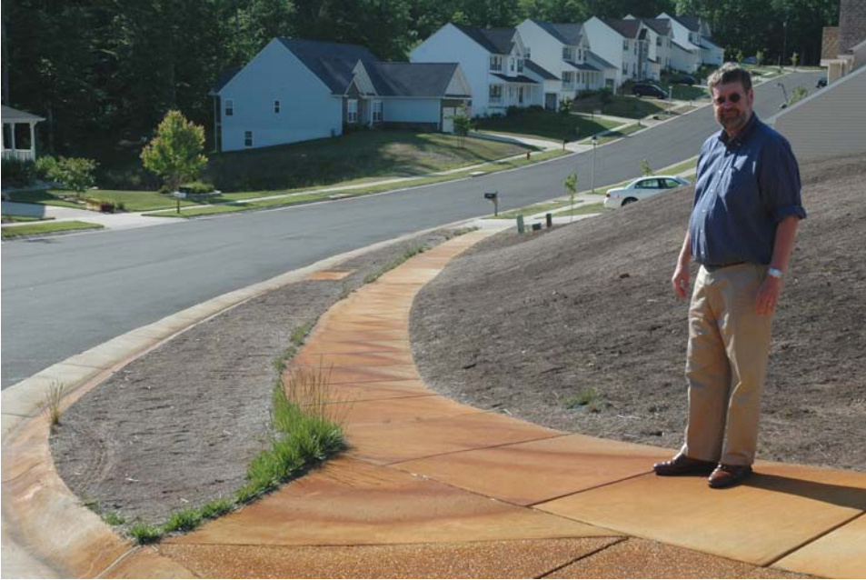
Lee Daniels, soil scientist and reclamation expert from Virginia Tech is shown standing on discolored side walk around house at the corner of Great Oaks Lane and Hickory Court. Grass is growing along the edge of the concrete probably because of the liming effect of the concrete.
