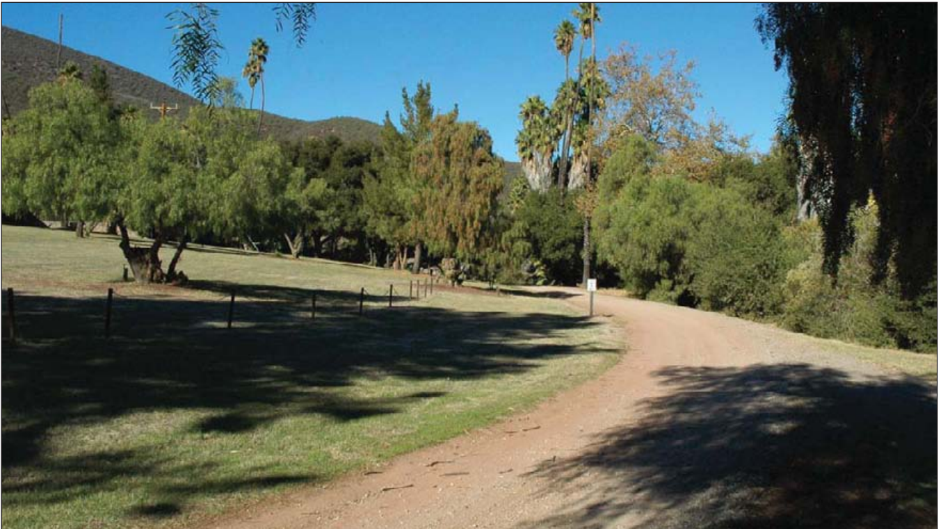
Photo: Internal road looking north heading toward the exit of the Project Site.
