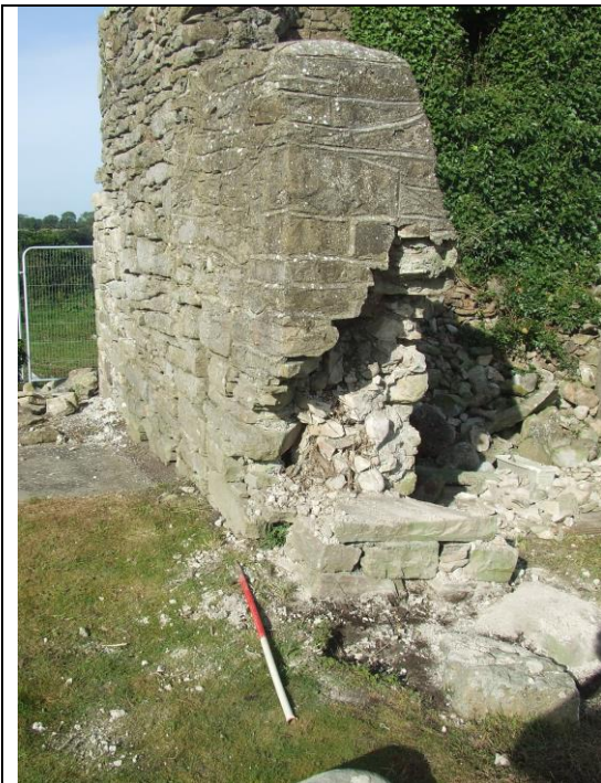
Plate 7 Bulkhead in southern wall prior to repair.
