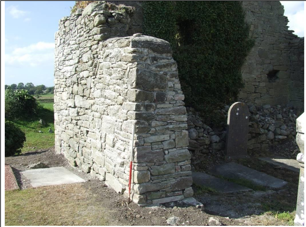
Plate 9 Repaired Bulkhead in southern wall, facing northwest.
