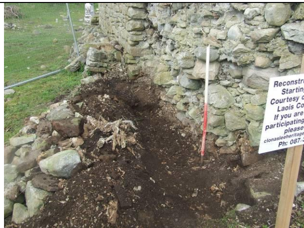
Plate 3 Excavation area at west elevation of west gable, facing north.
