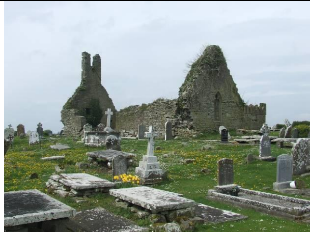
Plate 1 Showing Kilmanman Church prior to works taking place, facing NW.
