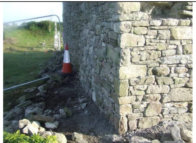
Plate 4 Repaired west gable wall, facing north.
