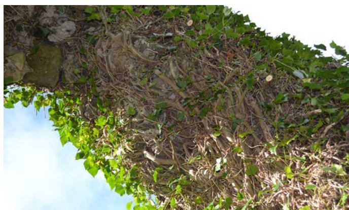
Detail of underside of chancel arch after trimming.
