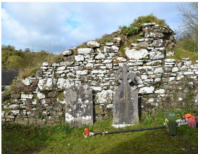
View of north wall masonry from nave.
