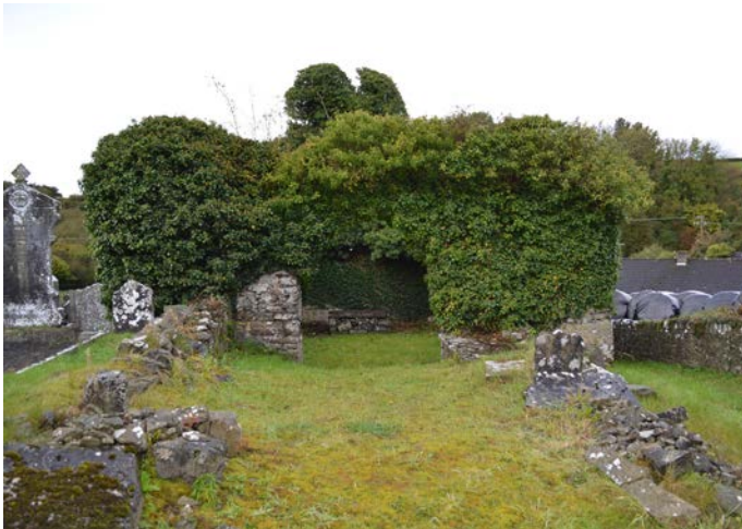
View of the east end prior to trimming.
