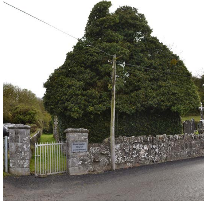
West gable prior to trimming.
