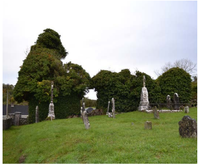
General view from the south prior to trimming.
