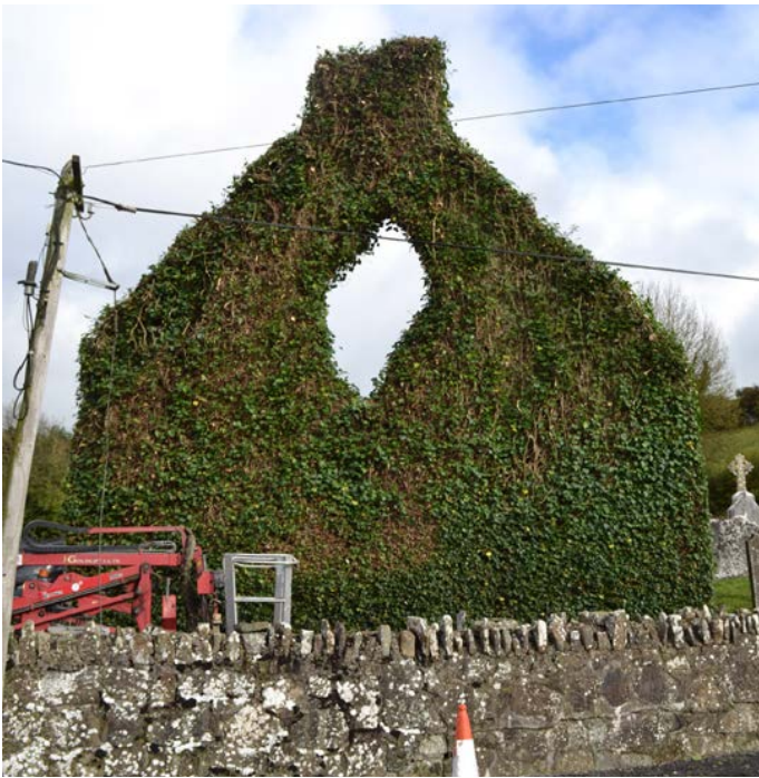
West gable after trimming.
