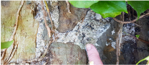
West gable wall - internal Significant ivy growth around arch window with roots embedded in masonry
