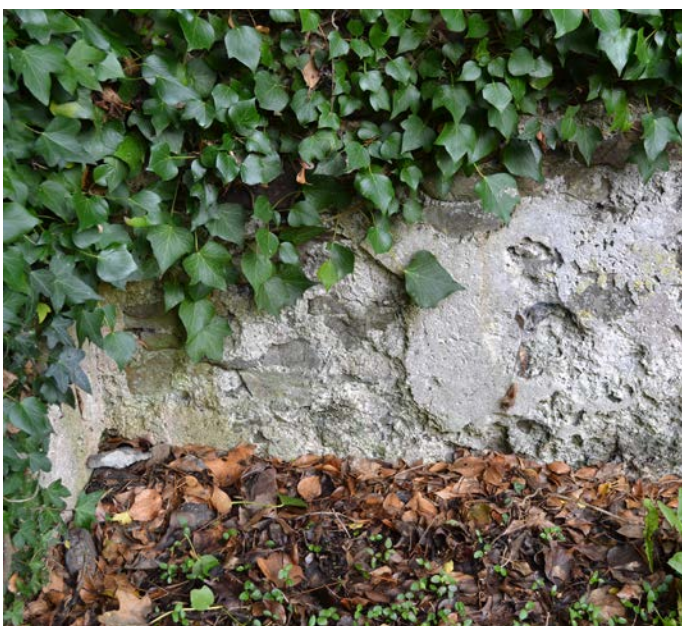
Surviving lime plaster in north west corner of nave.
