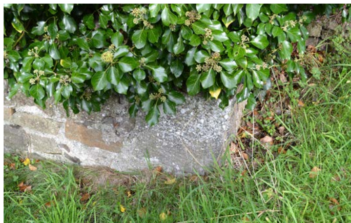
Detail of sandstone quoin at south east corner of nave.
