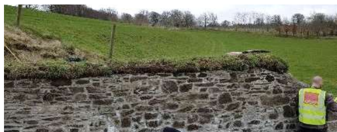
Example of a completed soft capping to wall head.
