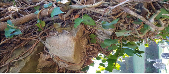
Pictures of ivy to inside edges of west window- Stones are being held in place by ivy therefore ivy removal needs to be carried out by stone mason and stones identified and referenced as dismantled
