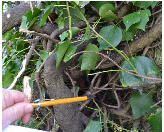
Close up of ivy stems on west gable after trimming.
