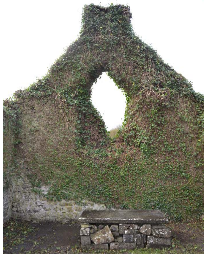
West gable from the nave after trimming.
