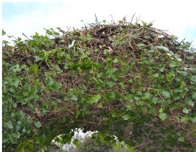
Detail of chancel arch from nave after trimming.
