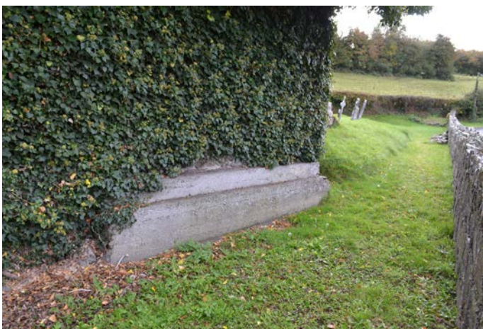
Concrete underpinning to west gable.
