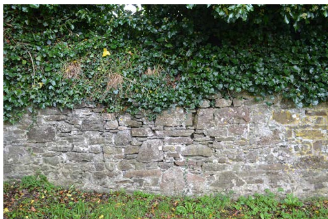
Detail of south wall of nave, interior view, showing uncoursed rubble stone pattern.
