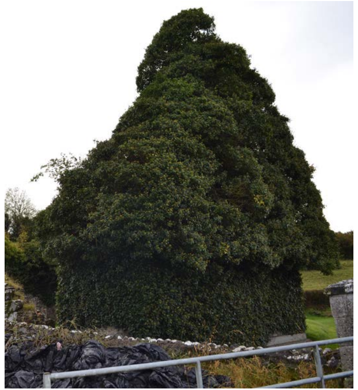
General view from north west prior to trimming.
