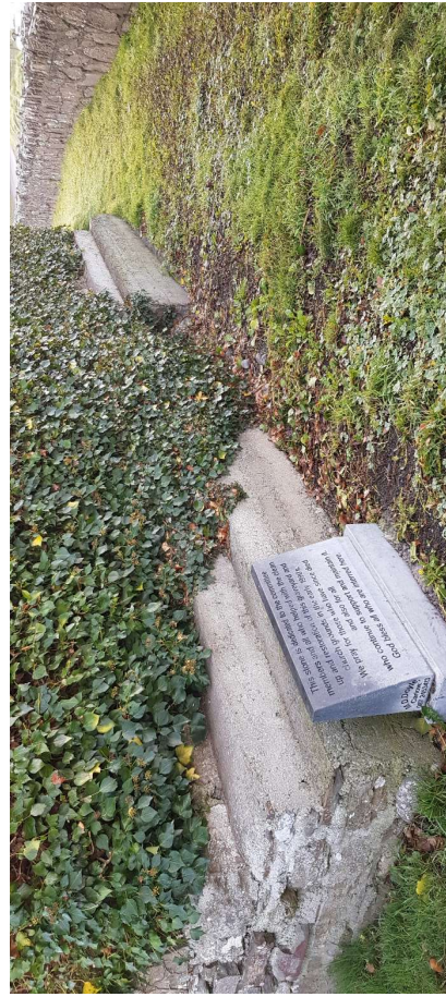
Rendered Masonry stepped plinth at external base of West gable
