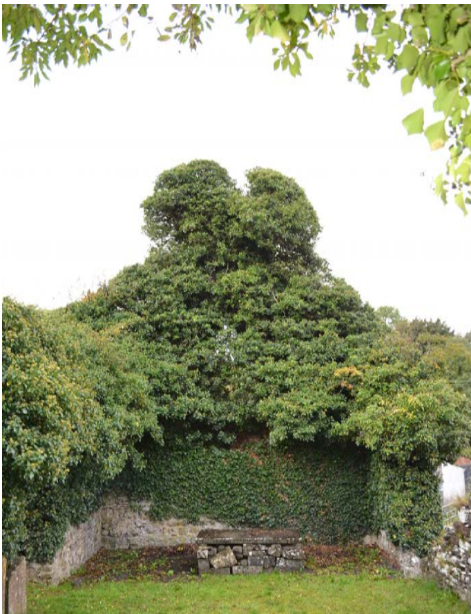
West gable from the nave before trimming.
