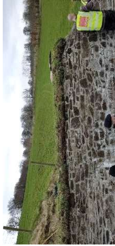
Below image, completed soft capping to wall head is shown.
