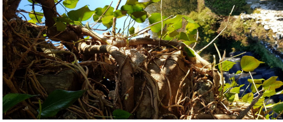
Pictures of ivy to inside edges of west window- Stones are being held in place by ivy therefore ivy removal needs to be carried out by stone mason and stones identified and referenced as dismantled
