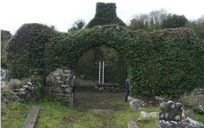
View of chancel arch from the east after trimming.
