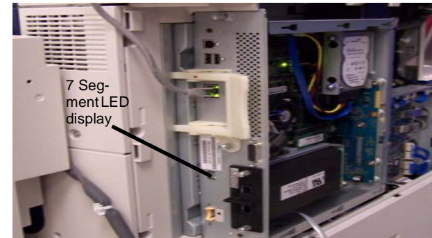
Figure 1 SBC 7-segment LED Location
