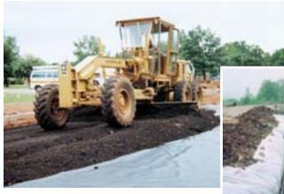
Left and inset: TerraTex SD Non-woven Geotextile (inset) from Hanes Geo Components aids in the filtration of water in highway edge drain applications, while TerraTex SD Woven
