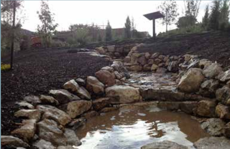
By utilizing slope and natural stone to slow down and manage water, traditional “Zuni bowls” and gabions are used throughout the garden. Photo by Clayton Bass
