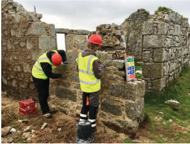
Repairing the walls of the Isolation Hospital. © Charlie Smith
