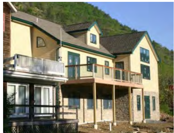
The new LGNC visitor and education center
