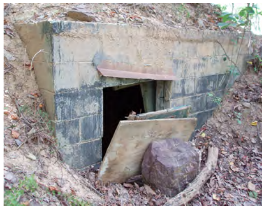
Block building near Lehigh Tunnel
