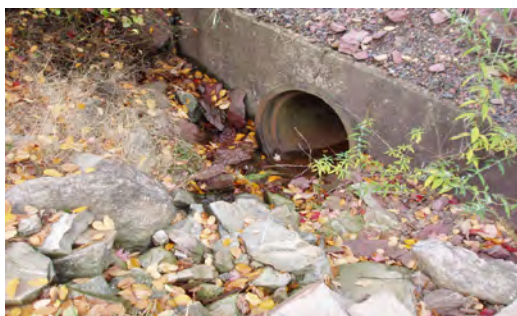
Stormwater culvert
