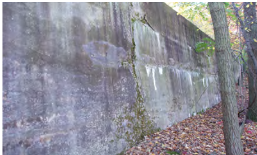
Concrete and wood retaining walls (above and right top and bottom)
