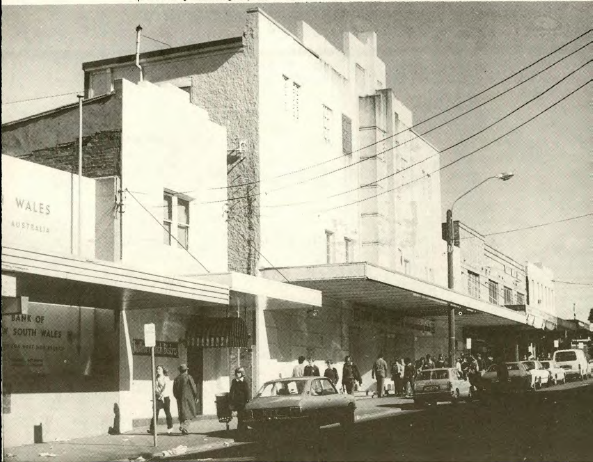
Arcadia Theatre, western end of Victoria Avenue, built 1915, modernised 1936. (Photo by Willoughby Municipal Library, taken June 1981.)
