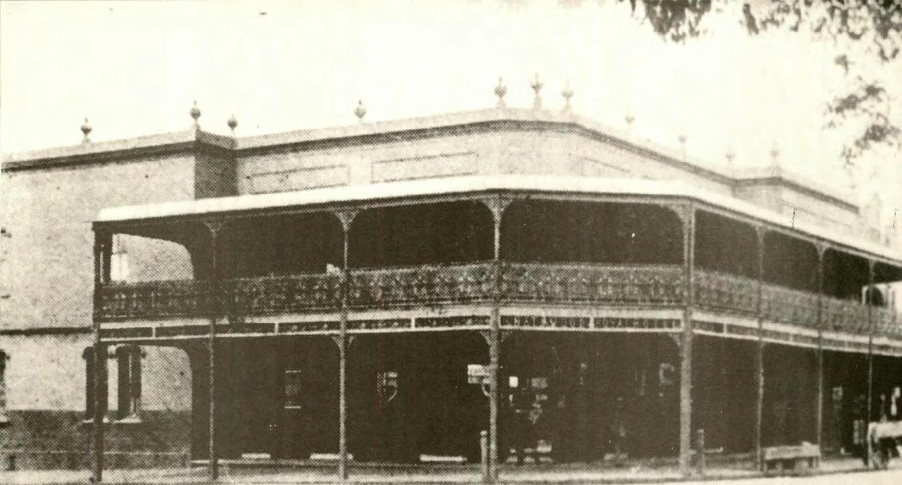
Royal Hotel (Sharland's), Gordon Road, now Pacific Highway. (Horse trough, iron lace around balcony and wooden posts supporting balcony.) (Photo by courtesy of Willoughby Municipal Library)
