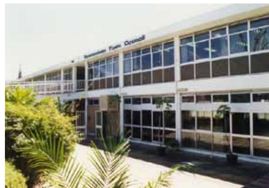
Bassendean Town Council administration building, 1988 (BLHC P800)
