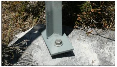
Figure 2. Modified star iron used to fix corner posts of exclosure. 8 x 60 mm threaded rod was held in rock by Sika AnchorFix chemical anchor into holes drilled with a cordless rotary hammer TE 6-A36-AVR.
