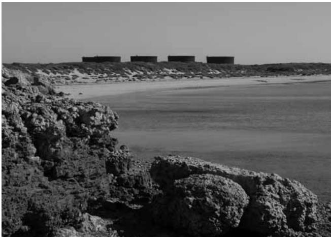
Terminal tanks on the east coast of Barrow Island Nature Reserve near Town Point – Photo Fran Stanley (DEC)
