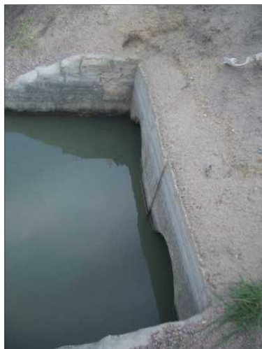
Plate 1. Existing Culvert Structure on Coolgardie-Esperance Highway
