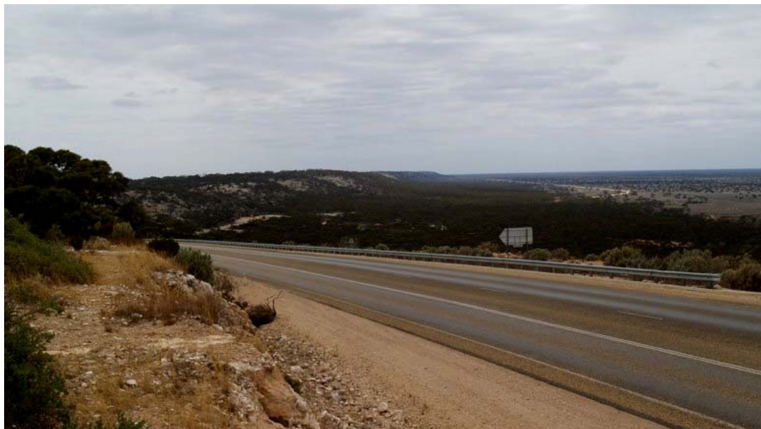
Photo 7 Hampton Tableland at Madura Pass, Eyre Highway
