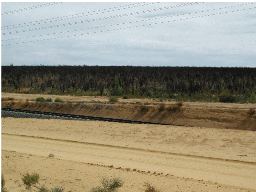
Figure 20: the Perth-Kalgoorlie railway line passing through an area of burnt shrubland.
