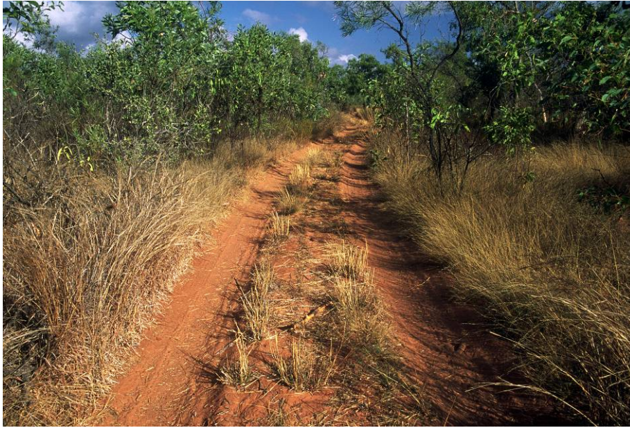
Photo 12. A low impact vehicle track on Dampier Peninsula created without removing topsoil (September 2002).
