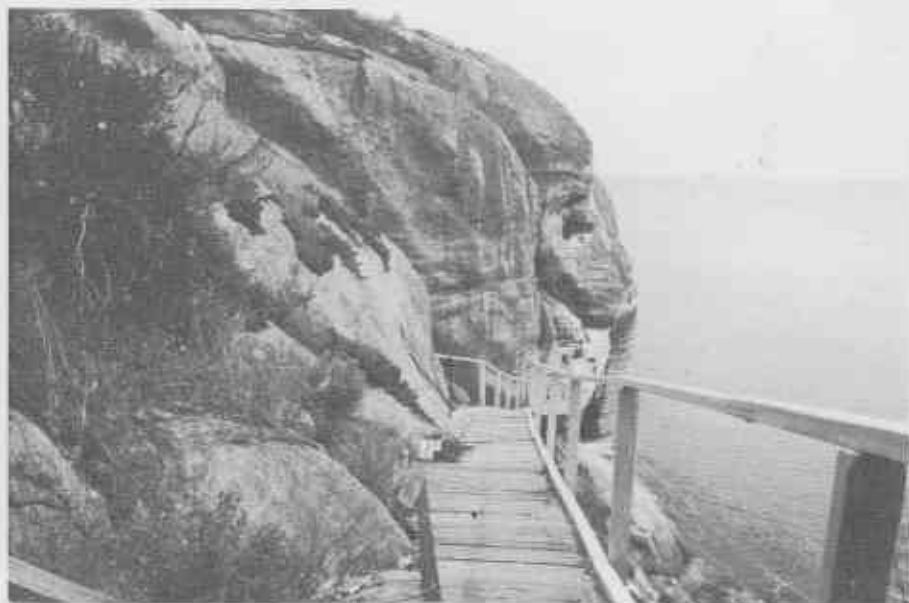
PLATE 8. Walkway from the wharf recently constructed on the island's north-eastern side.
