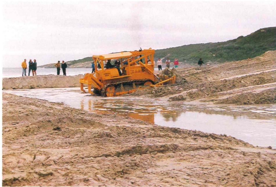
Wilson Inlet. Excavating the cut through the bar, 14 June 1988.
