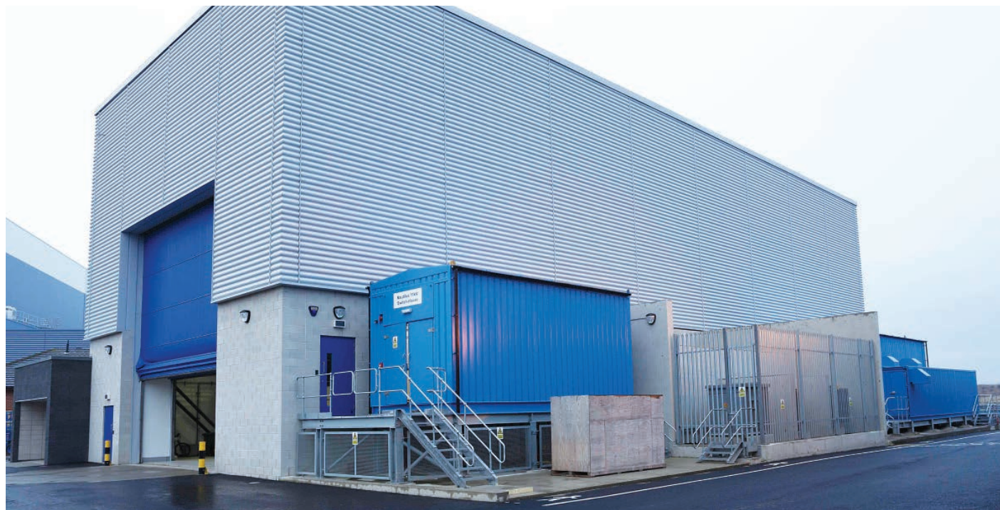
The test hall houses the 3 MW turbine drive train test rig.
