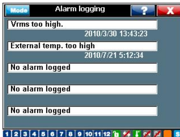
Figure 50: Bank monitoring alarm logging
