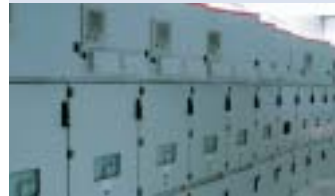
ABB's UniGear ZS1 panel is an extremely versatile platform for medium-voltage switchgear in the 12-24 kilovolt range.
