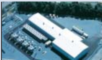
ABB's unique HVDC Light system is designed for underground or underwater power transmission. Its environmental benefits include no overhead power lines and a neutral electromagnetic field.
