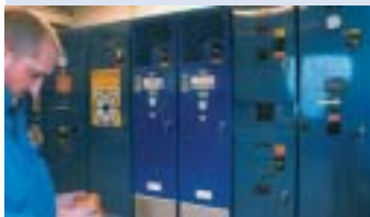
ABB's drives sharply reduce energy consumption and cut costs.
