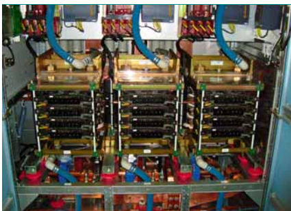
7 Inverter unit of ACS6000 frequency converter
