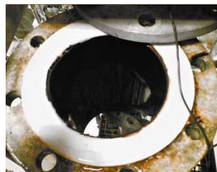
6 Coated magnetic flow meter in a pulp and paper application
