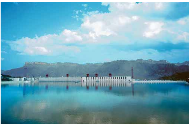
4 The Three Gorges hydroelectric power plant in China
