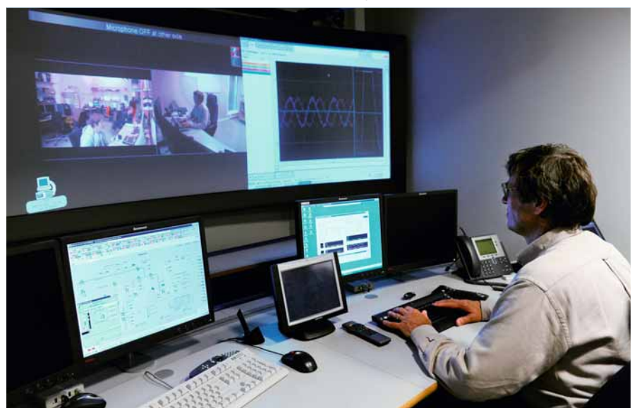
1 ABB-Shell collaboration room – an example of an integrated operations center
