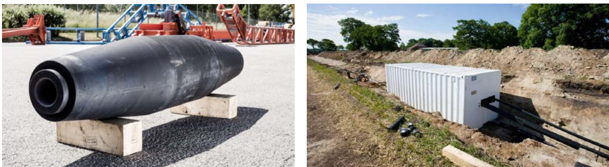
Figure 5. (a) A 525 kV rubber body, (b) A specifically built container for underground cable jointing.
