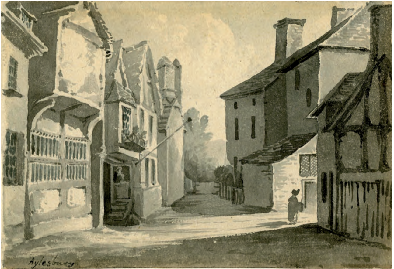
Figure 83. Watercolour of c.1810–30 by Amelia Long looking east along an alleyway which runs along the course of the former hillfort bank. The medieval King's Head on the left, would have been constructed on the site of its bank. It is possible that the entrance into its courtyard (visible on the left) could be on the site of one of the hillfort's entrances. (Reproduced courtesy Buckinghamshire County Museum ref AYBCM 1968.126.3).
