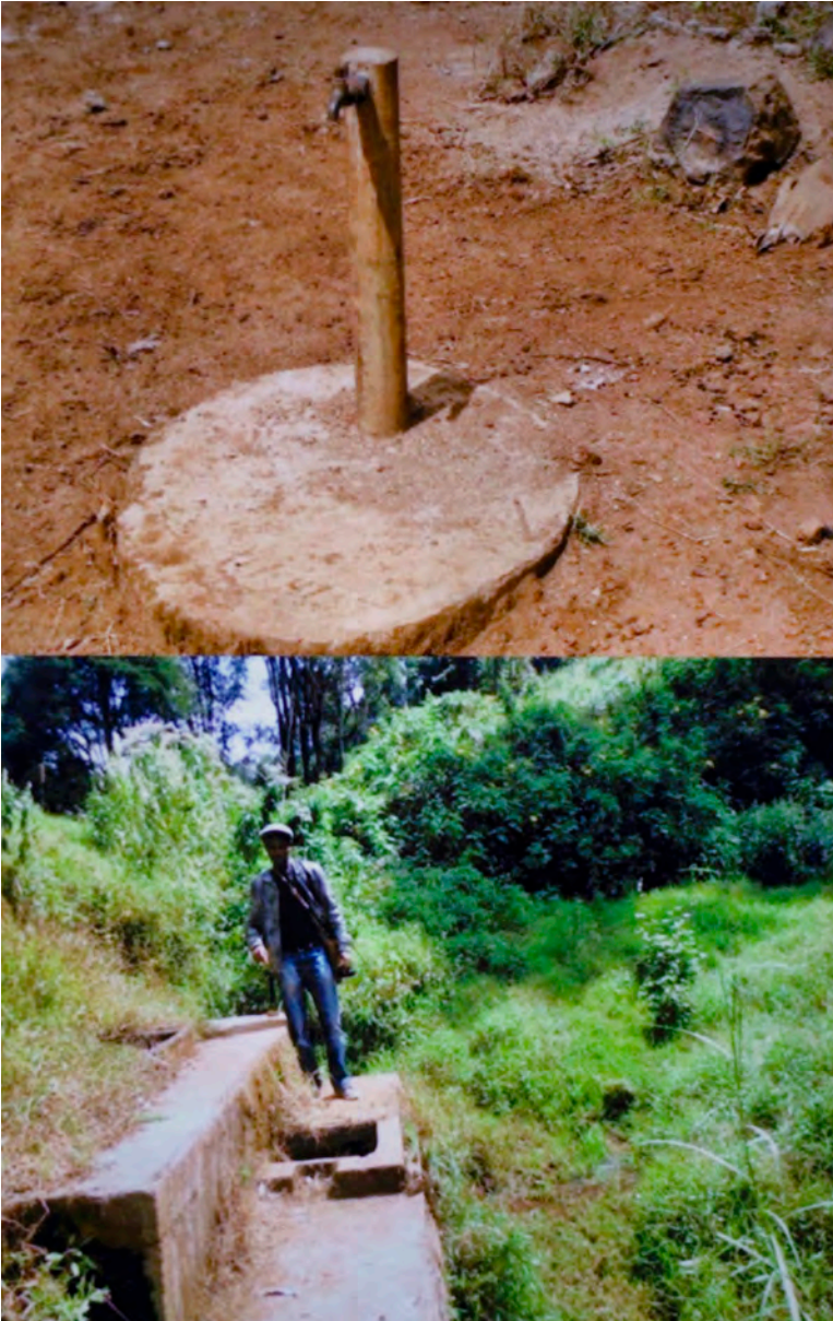
FIGURE 7.2. Dilapidated Water Catchment Tank and Abandoned Stand Tap Due to Poor Management in Ngarum-Ndu Municipality, Rural North-West Cameroon. Photo by Henry Bikiwibili Tantoh.
