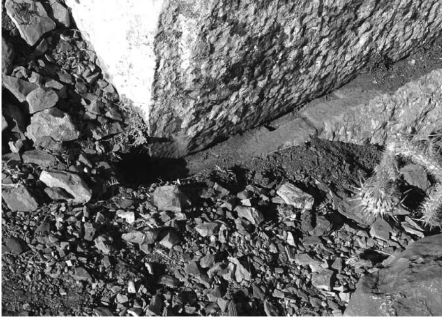
Figure 5. Rhodes, Mt Atavyros, Sanctuary of Zeus. Northern building: detail of the north wall with bevelled corner and Π-shaped metal clamp (photograph by M. Livadiotti).
