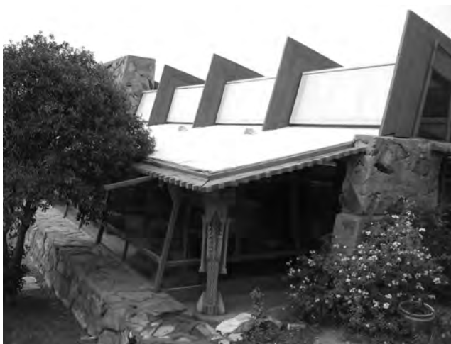
FIGURE 28.10 Taliesin West in Scottsdale—when Wright set out to design and build Taliesin West, his goal was to integrate the structures with the “nature” of the desert, its soul, and with the desert’s nature, its physical characteristics. (From Lucas, S.A., Taliesin West: In the Realm of Ideas , The Frank Lloyd Wright Foundation, Scottsdale, AZ, 1993.)
