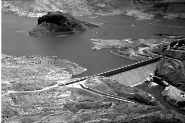
FIGURE 26.6 Elephant Butte Dam. (Courtesy of the U.S. Bureau of Reclamation.)
