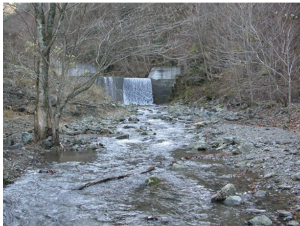
Fig. 12.6 Erosion control dams in mountain streams
