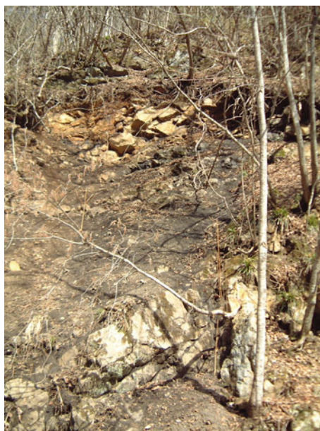
Fig. 6.16 Small landslide on the lower side slope
