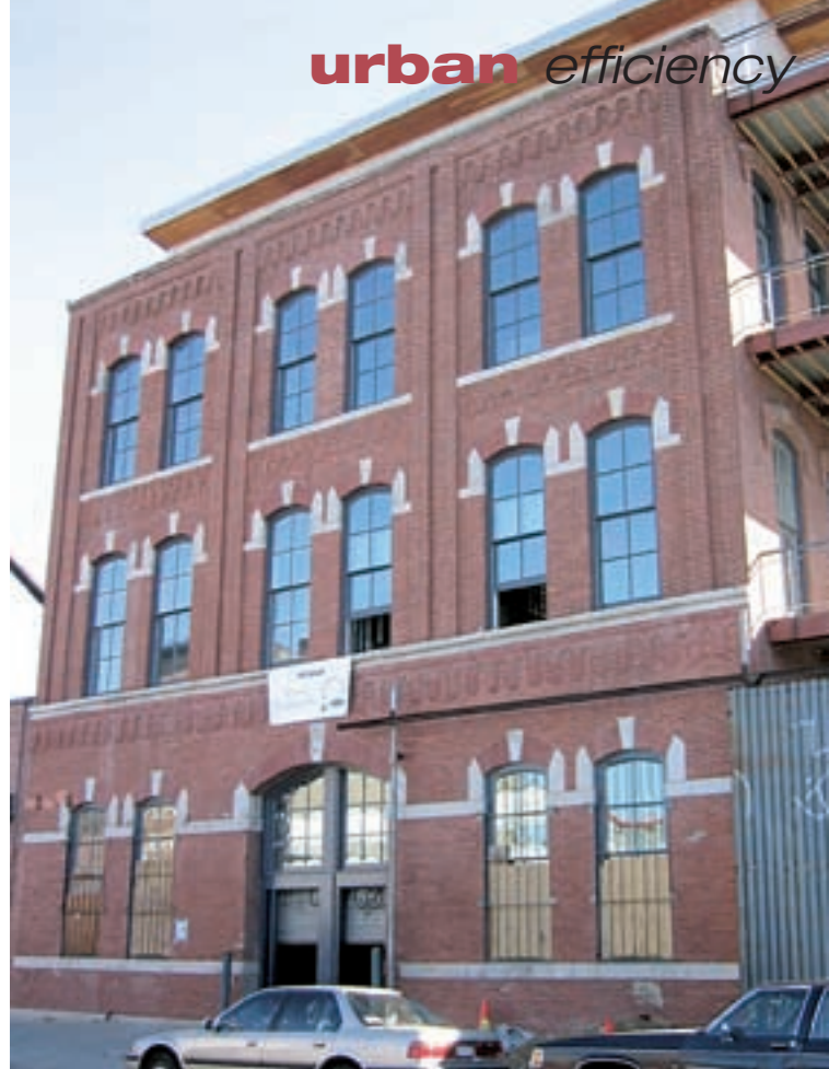
The new, energy-efficient icehouse nears completion.
