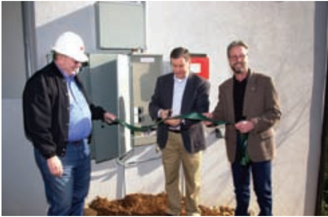
Mike Glancy from local utility Entergy Arkansas, Arkansas Renewable Energy Association president Bob Harp, and contractor William Ball cut the ribbon upon commissioning the net metering system.
