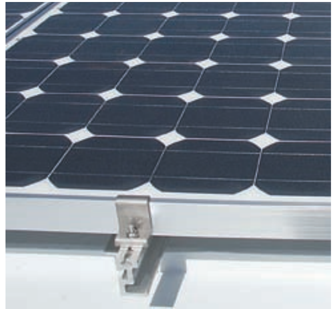
Clamps at the ends of the Power Rail secure the PV panels along their outside edges.
