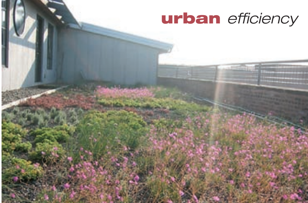
Besides lending a lush, colorful landscape to what would otherwise be a barren surface, the icehouse’s green roofs provide the building with additional insulation, act as evaporative coolers, and help manage water runoff.
