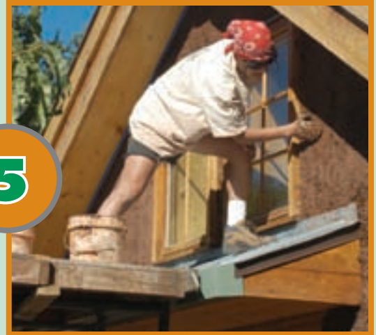
Satomi Lander of Kingston, New Mexico, demonstrates the artful technique of applying earthen plaster to this straw bale home.
