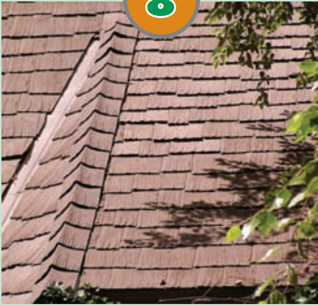
Eco-shake roofing shingles are made from post-industrial recycled PVC and 100 percent reclaimed wood fibers.
