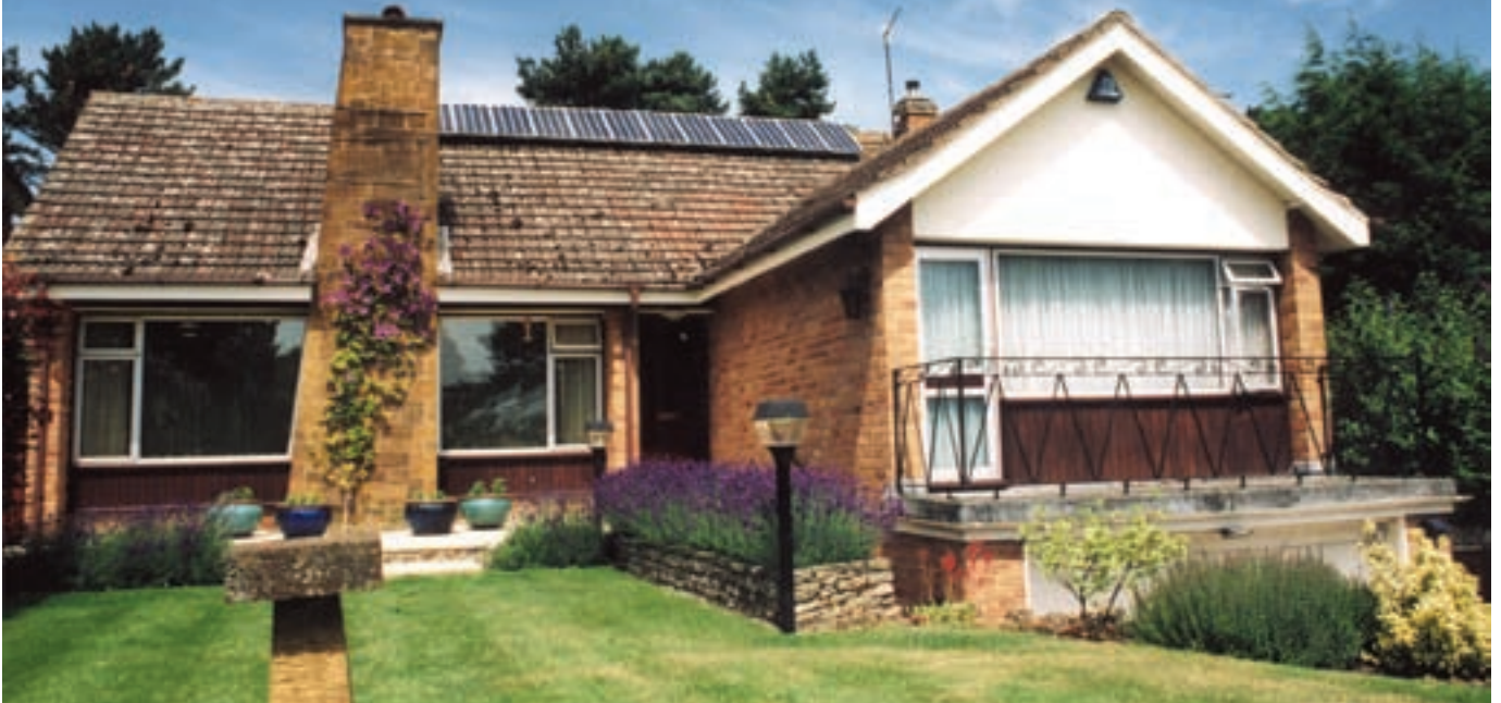
A 1,020-watt PV array on the roof of Anthony Skelton's house in Leek Wootton, United Kingdom, is only half of his total solar array.
