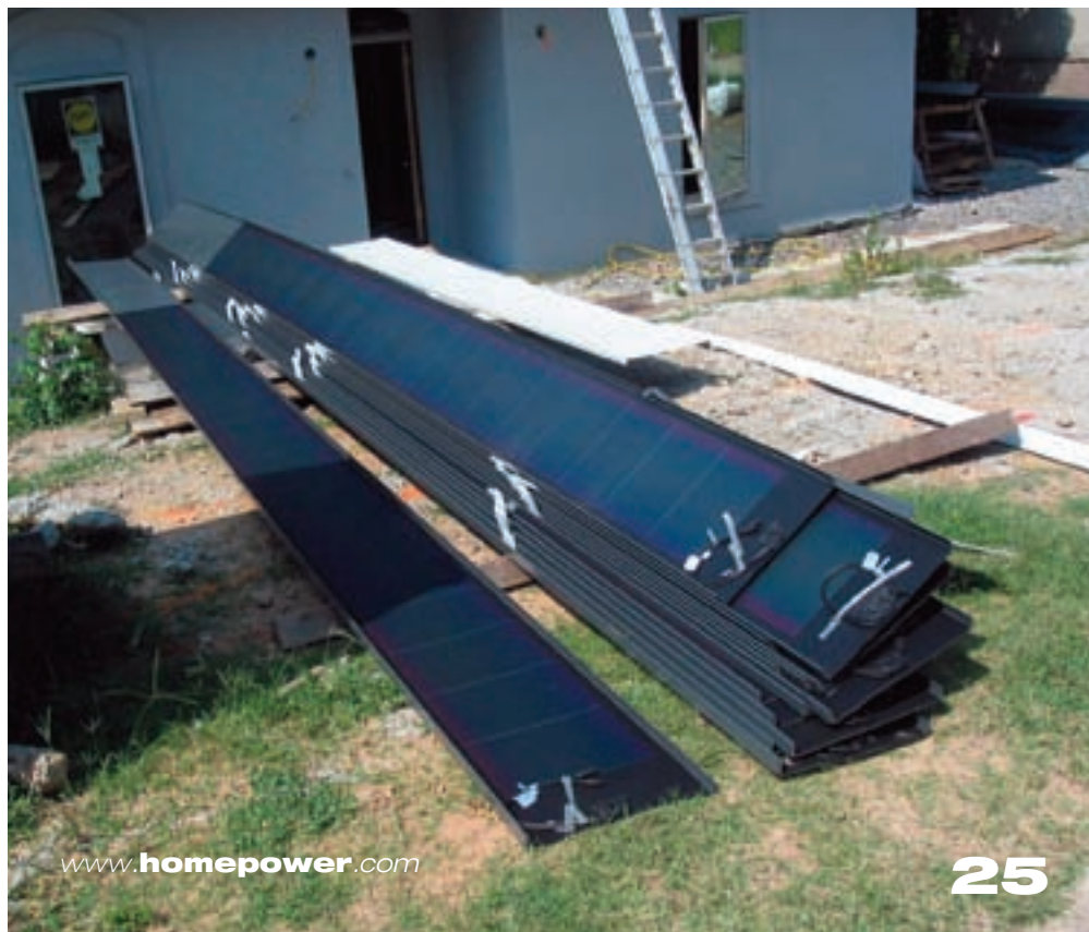
PV laminated roof panels ready to go up on the roof.
