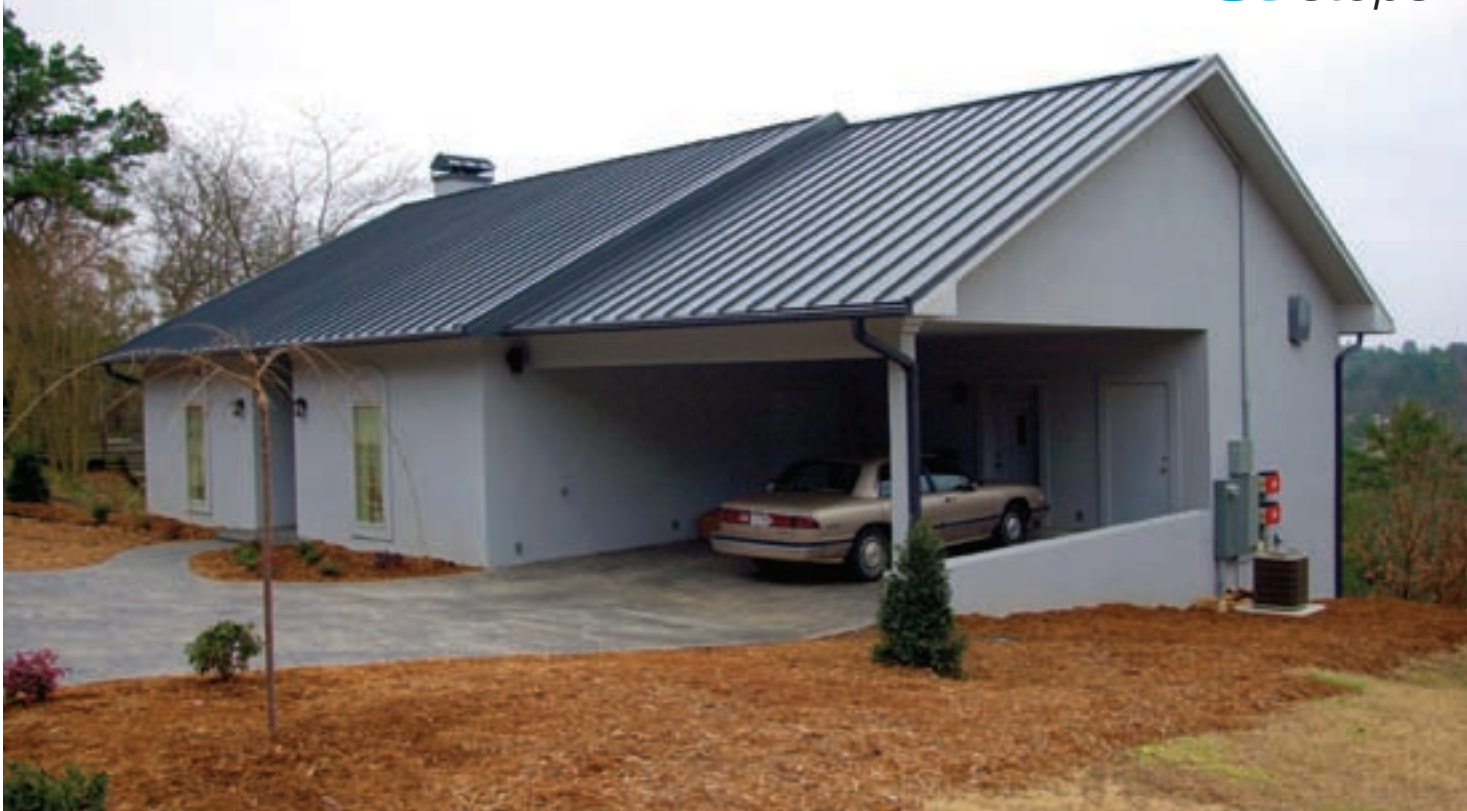
This home looks like any other, except it's solar powered. Inverters are visible on the right side of the building.
