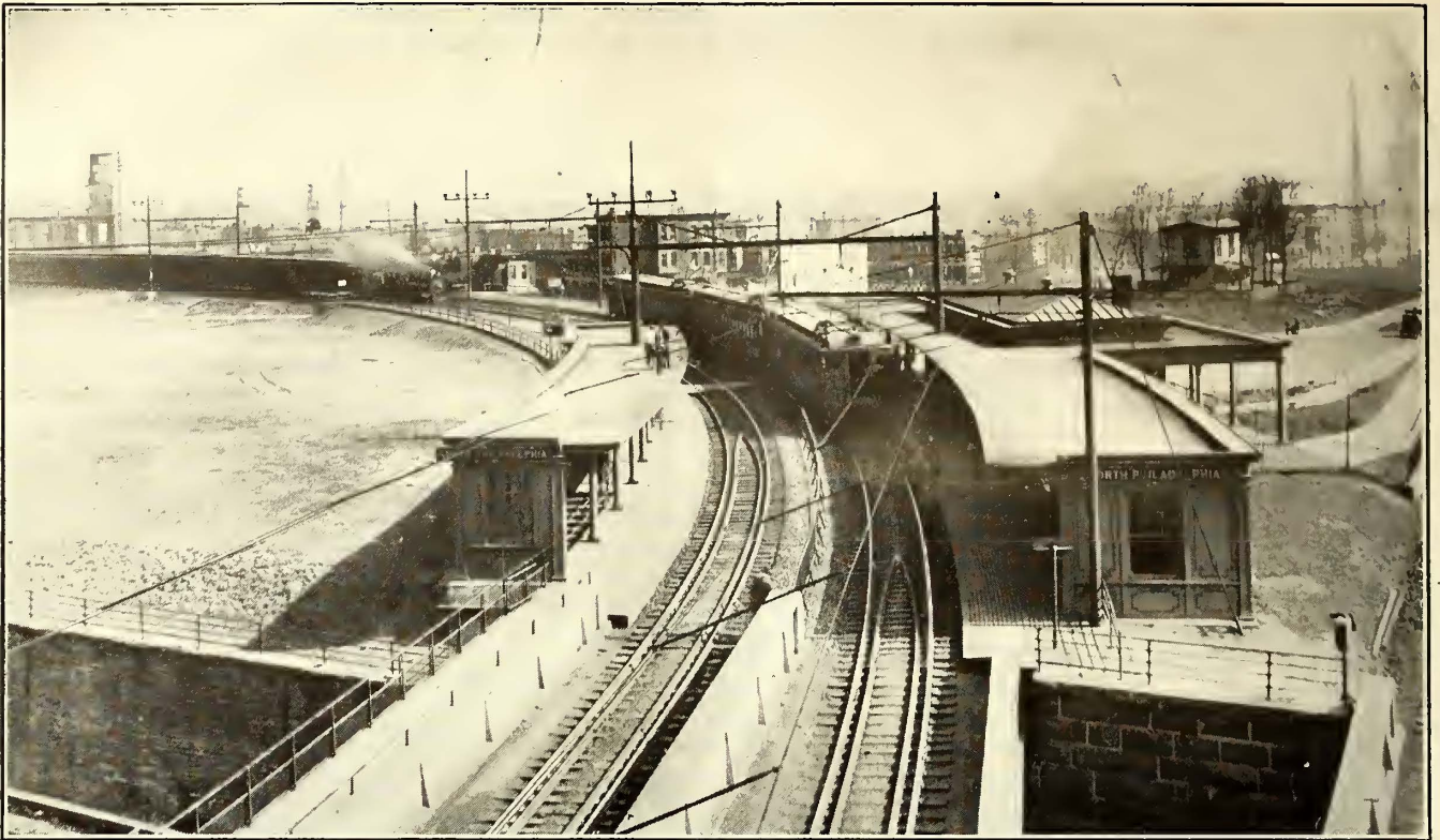
VIEW FROM SIGNAL BRIDGE AT NORTH PHILADELPHIA SHOWING TYPICAL METHODS OF CATENARY SUPPORT
