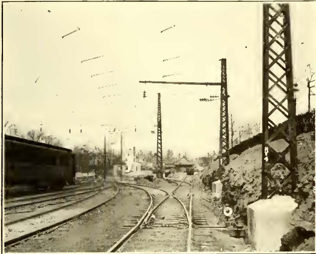
CHESTNUT HILL YARD SHOWING LATTICED POLES SUPPORTING CATENARY STRUCTURE
