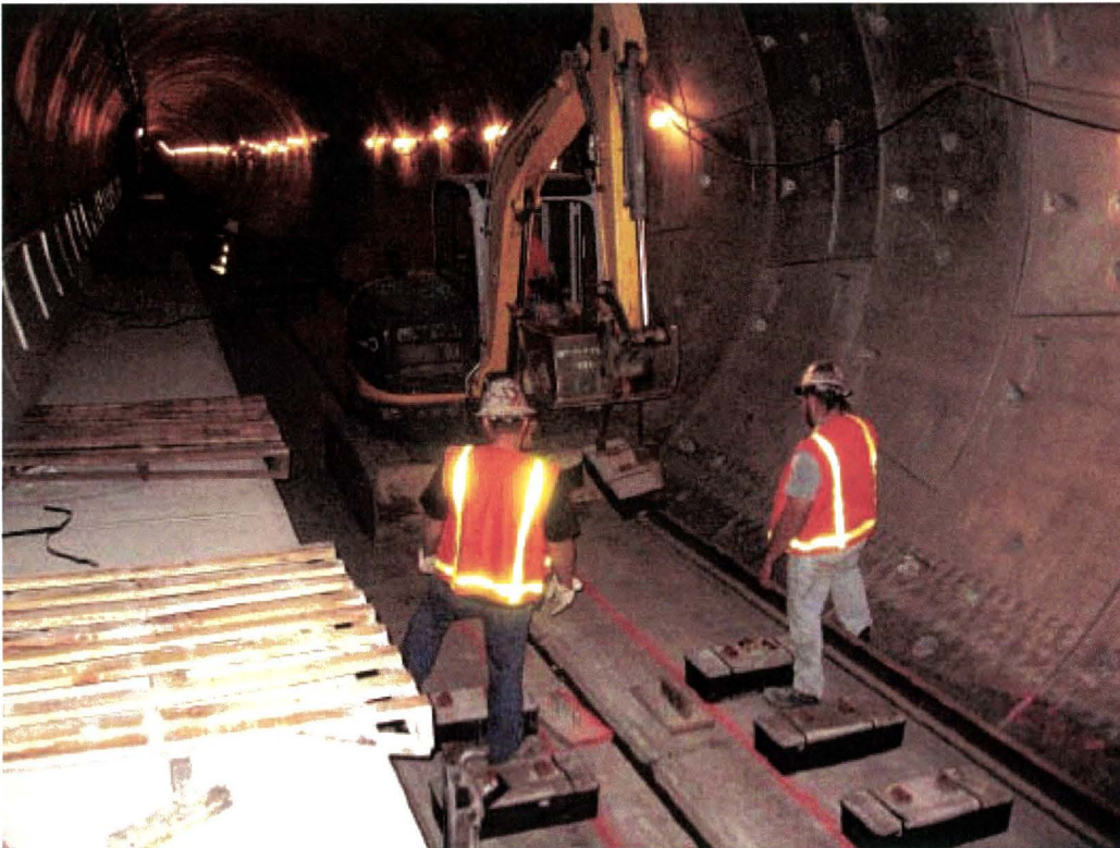
Installation of LTV Blocks within the Tunnels Prior to Rail Installation
