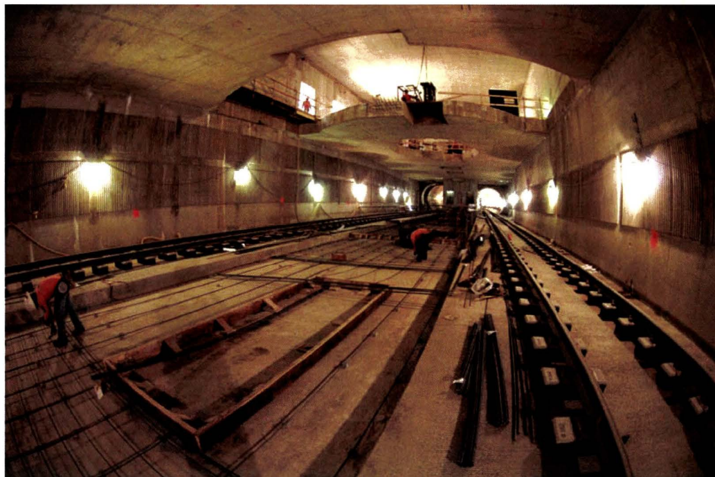
Soto Station Construction
