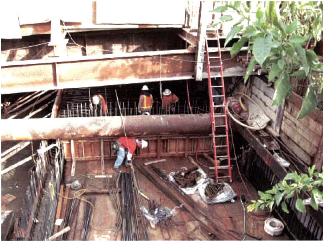
Roof Rebar Installation at Boyle/Heights Mariachi Plaza Station
