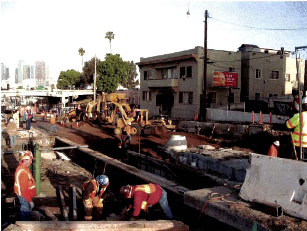
Earth Backfill over the Underground Structures
