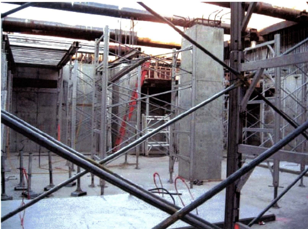
Construction of Boyle Heights Mariachi Plaza Station
