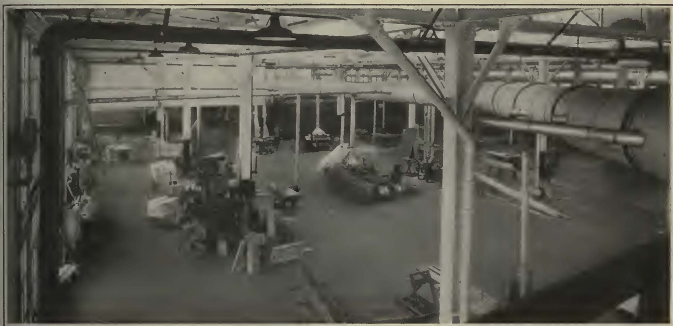
Noteworthy Features of the Wood Mill Are the Individual Motor Drives for All Tools and the Suction Dust Collecting System
