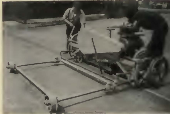
"Vulcan" Rail Joint Grinder
