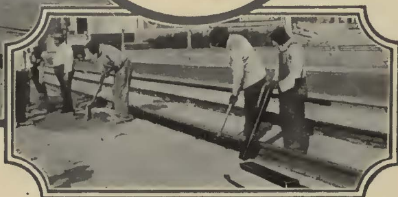
Gilbert Ave., Viaduct, Cincinnati, Ohio
