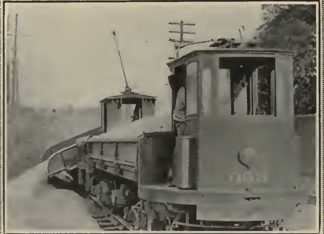
"Differential Two-Car Train. Trailer dumping load clear of trench."
