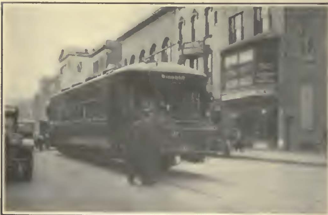
New Cars of This Type Have Reduced Energy Consumption on the Windsor Line of the York Railways
