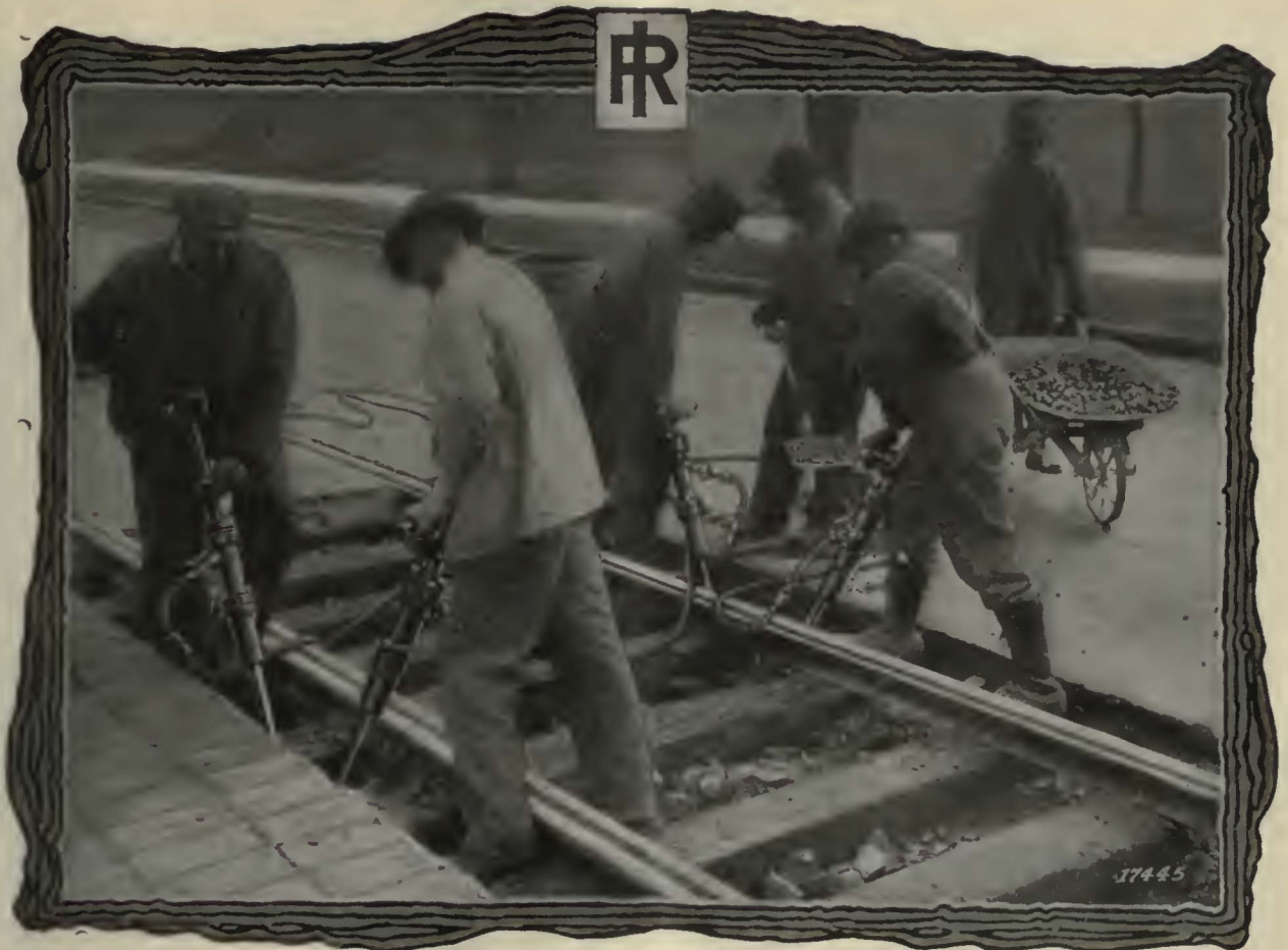
A four-tool pneumatic tamping gang at work on a track repair job
