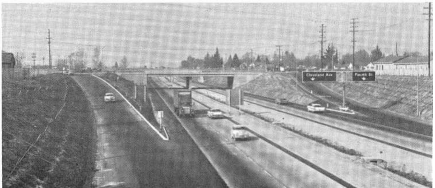
A view of the Madera Freeway looking north at the Fourth Street overcrossing. Landscaping of the freeway includes the planting of oleanders along the dividing strip and pyracantha on the slopes.
