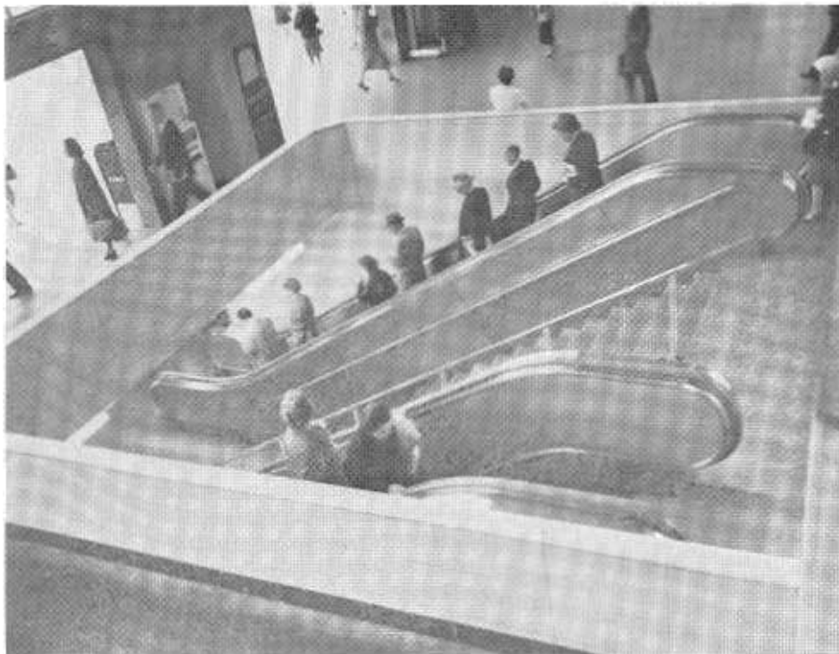
Included in the remodeling of the Transbay Transit Terminal in San Francisco was the installation of a new stairway flanked on both sides by escalators leading from the lobby to the mezzanine level.
