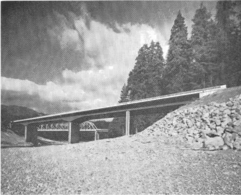
Bridges and freeway structures designed by the Division of Highways Bridge Department have been singled out for a number of awards in recent years. Last year this structure across the South Fork of the Eel River on US 101 (Redwood Highway) in Humboldt County was included among bridges judged most beautiful in national competition sponsored by the American Institute of Steel Construction.
