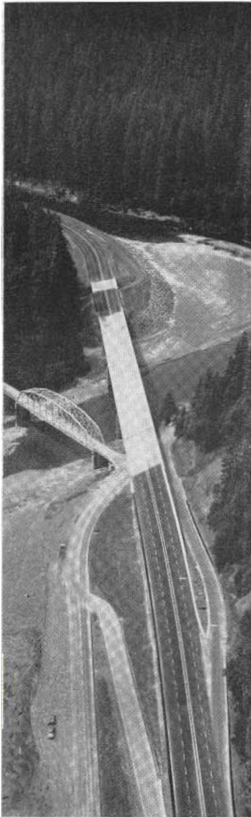
New freeway alignment of Redwood Highway (US 101) with prizewinning bridge over Eel River. Old bridge at left retained for access to redwood groves and parks.
