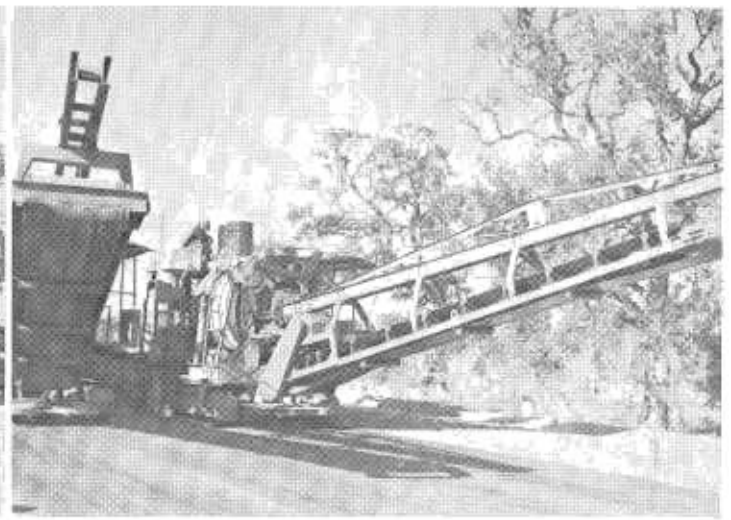
The belt conveyor discharge for the paving mixers.
