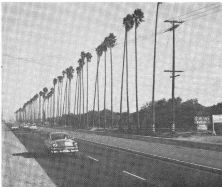
A view of the completed Lincoln Avenue widening project in Anaheim.
