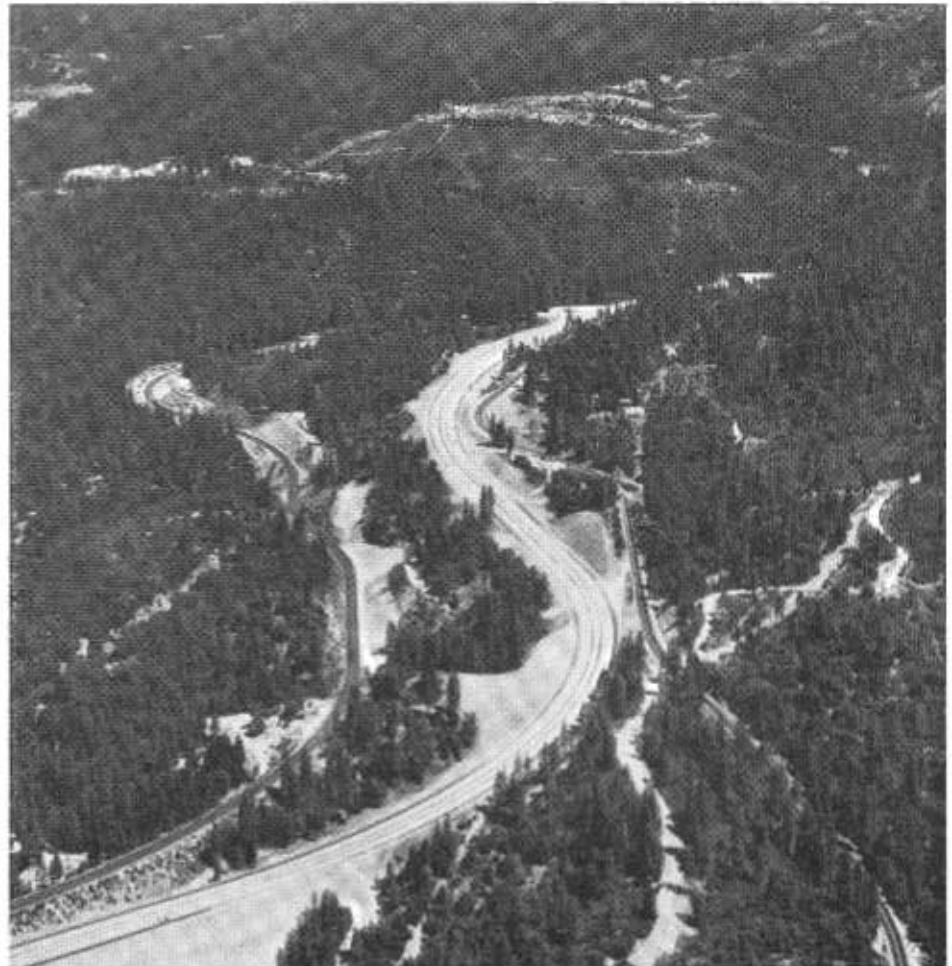
This new section of U. S. Highway 40 sweeps in graceful curves through the rugged terrain of the Sierra-Nevada east of Colfax. Several large-scale freeway projects were completed on this major Interstate Highway in 1959.
