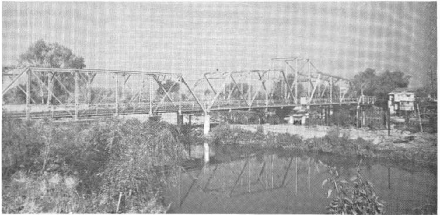
The original Grant Line Canal bridge completed by San Joaquin County in 1906. Although still standing, it is incapable of carrying heavy tonnage trucks.
