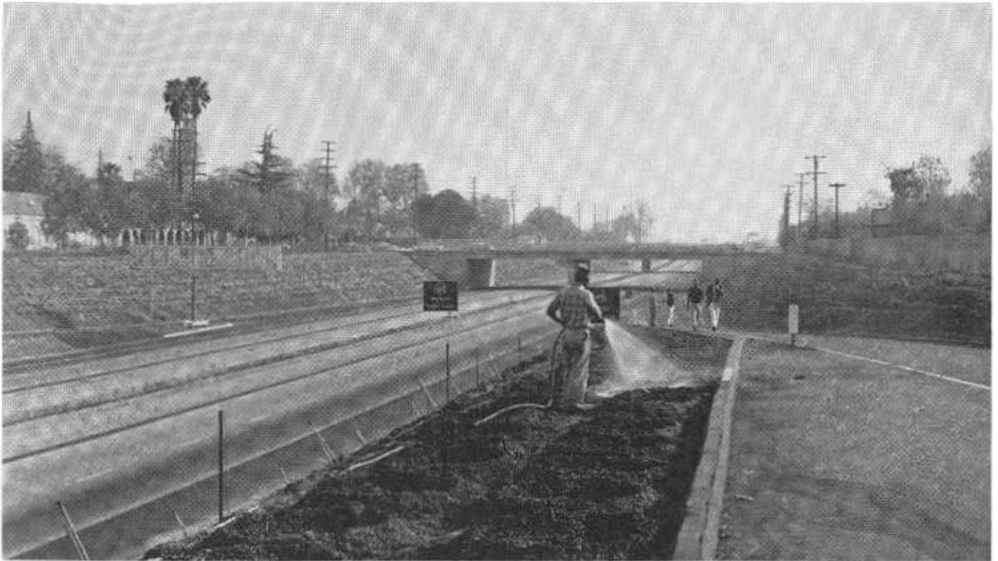
A low-lying species of pyracantha was planted on the slopes of the Madera Freeway to give an effective yet attractive ground cover.
