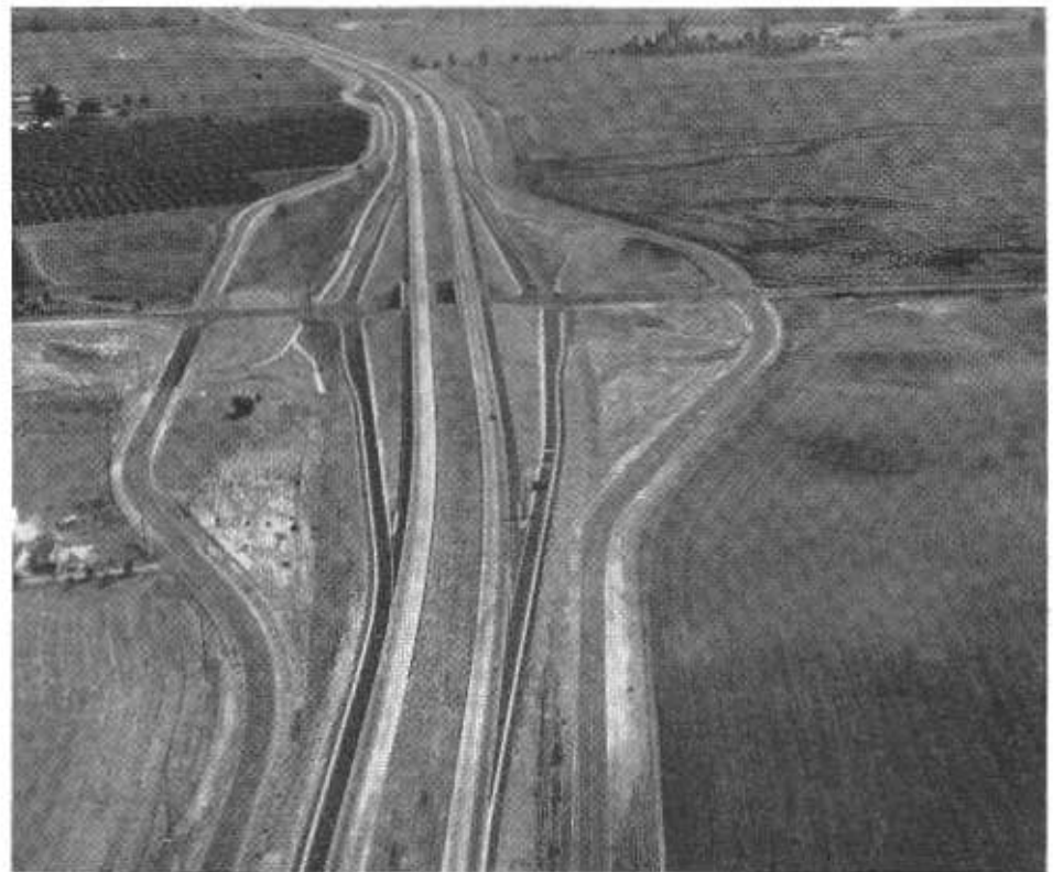
Another section of the San Diego Freeway in Orange County has been completed. This southward view shows the Niguel Road-El Toro Road Interchange.
