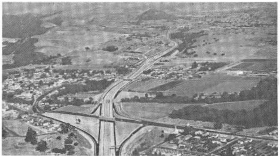
US 101 converted to full freeway through Arroyo Grande in San Luis Obispo County.
