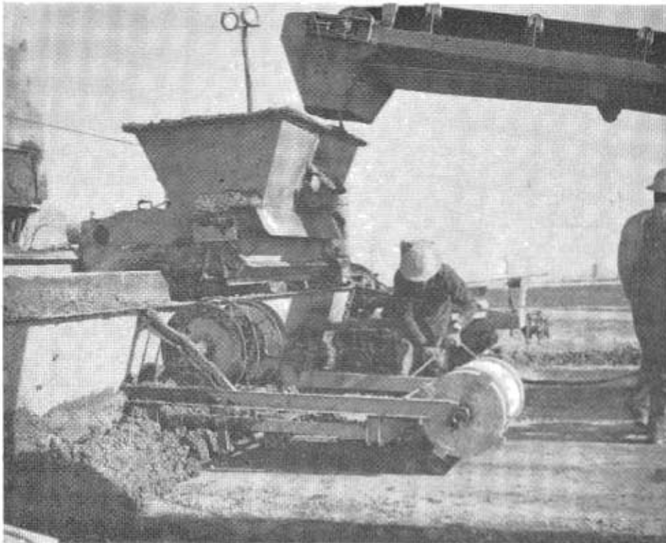
A device for installing reinforcing steel as tie bars across longitudinal weakened plane joints.
