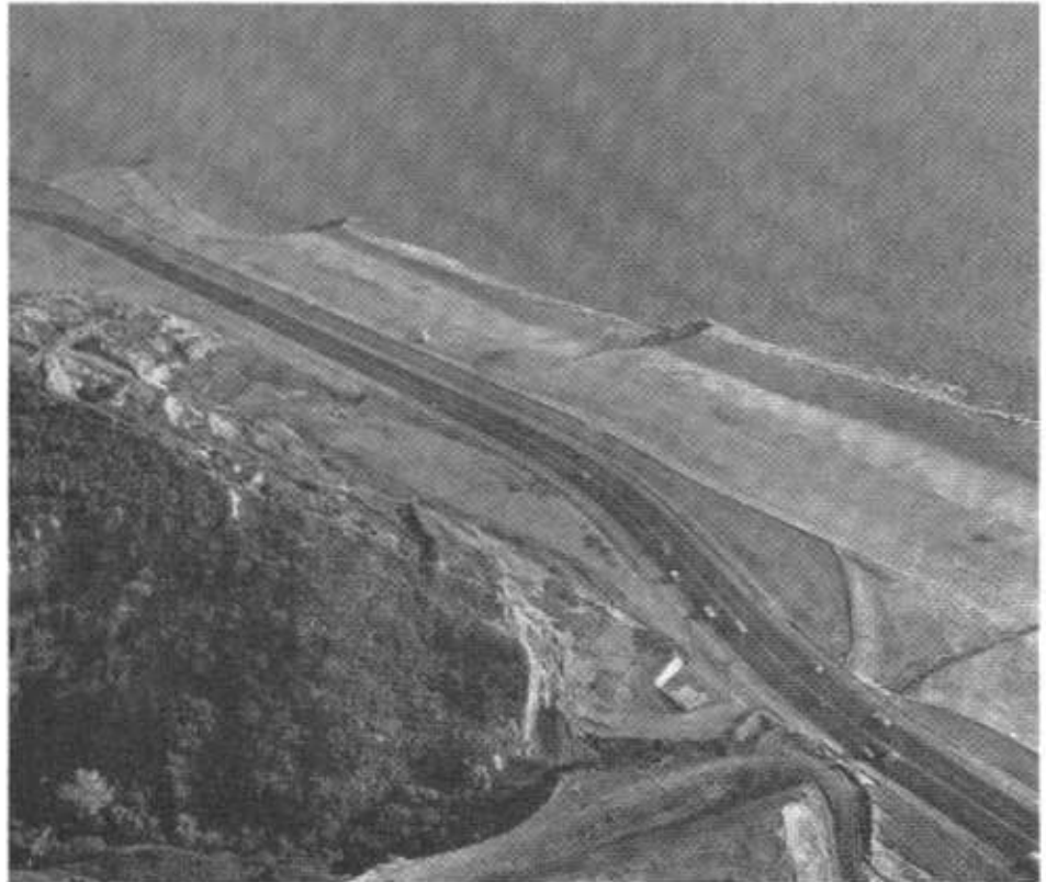
The relocation of a section of U.S. 101 Alternate in the Pacific Palisades slide area has been completed.
