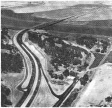
Modernization of section of Black Point Cutoff in Marin County and completion of the new Petaluma Creek bridge.
