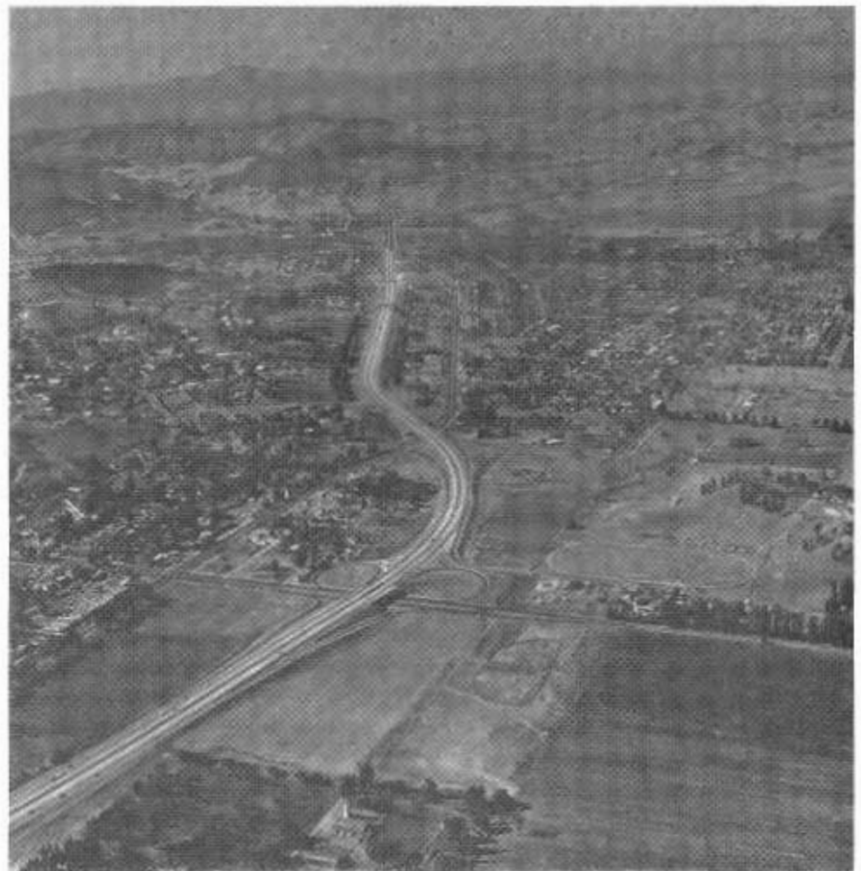
Looking west along a new section of the Ventura Freeway through the Woodland Hills area in the San Fernando Valley. In the foreground is the Topanga Avenue interchange.
