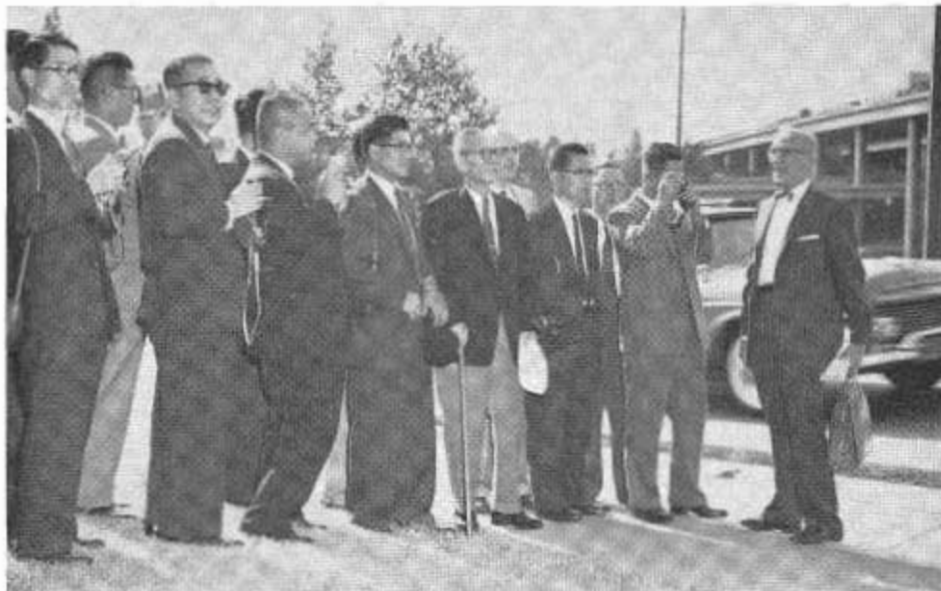
A group of engineers and officials from Japan visit the four-level grade separation in downtown Los Angeles. Standing at right is Ramsey Stobie of the Training Within Industry Corporation of Cleveland, Ohio, who led the group on their tour.
