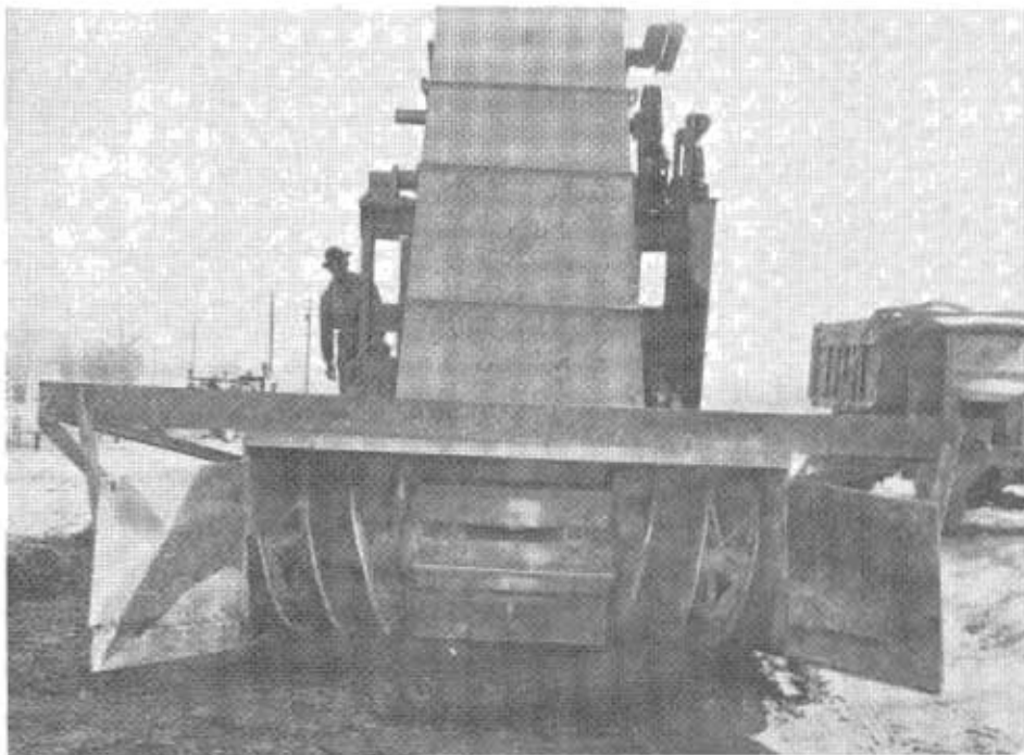
A front view of a mixer for cement-treated subgrade showing the bucket conveyor.
