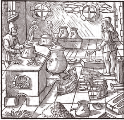
Fig. 7.26 Georgius Agricola, The extraction of sulphur from its ore , from De Re Metallica (Basel, 1556). Reprinted in Agricola & Hoover 1950 , p. 579.
