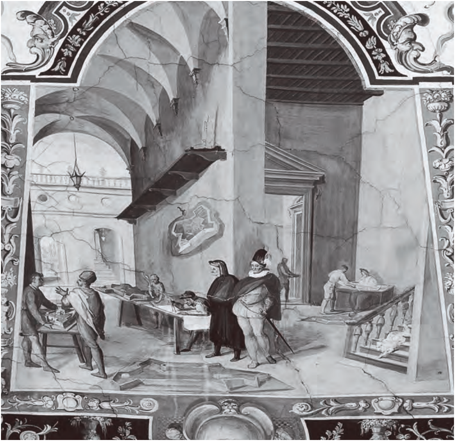
Fig. 8.4 Ludovico Buti, The Workshop of the Architect . Frescoed ceiling, 1588. Florence, Galleria degli Uffizi, room 23 (former 'armeria').
